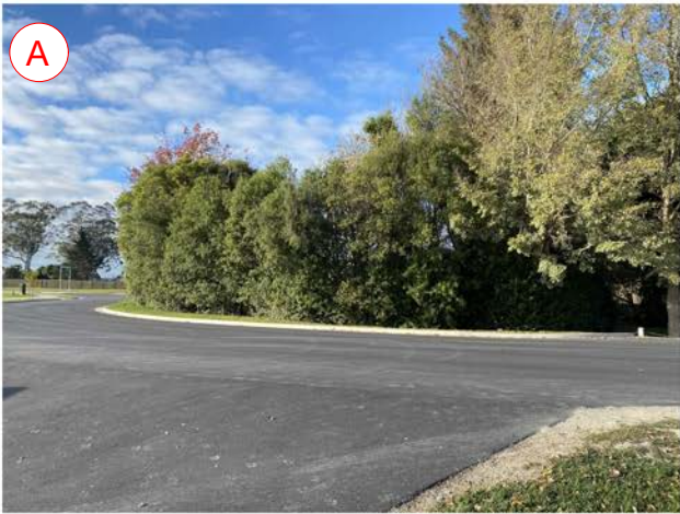
Sightlines around corner of Adderley Terrace are limited due to shrub vegetation. Vehicle sight lines are restricted. Shrub planting adjacent to the new footpath create CPTED issues (low visibility).
