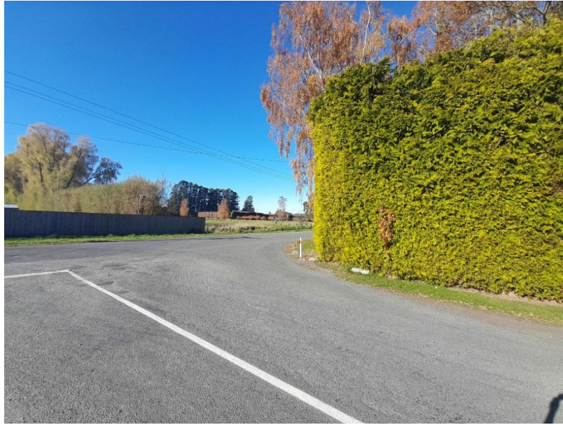
Figure 1: Baynons Road / Heywards Road intersection with restricted visibility
