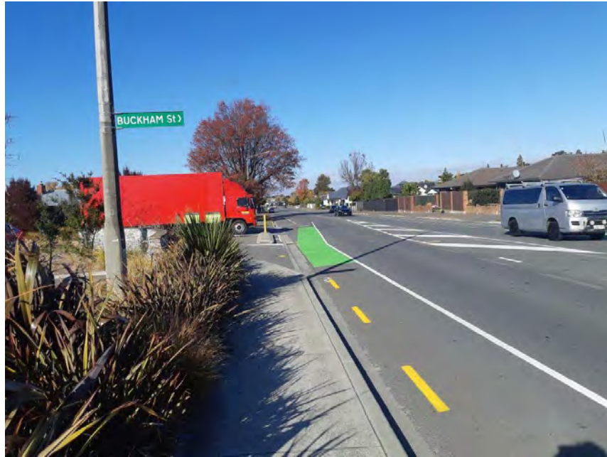
Figure 5. On-road cycle lane on Ivory Street.
