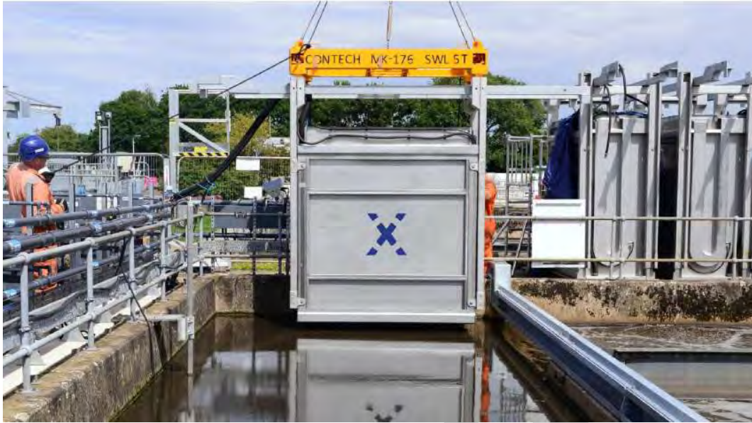
Figure 5 Example of an MABR module being installed (photo from Oxymem)
