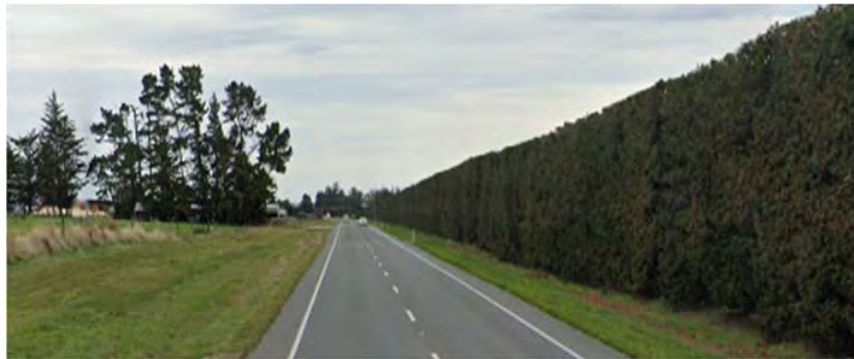
Figure 6. Shoulder widening.
