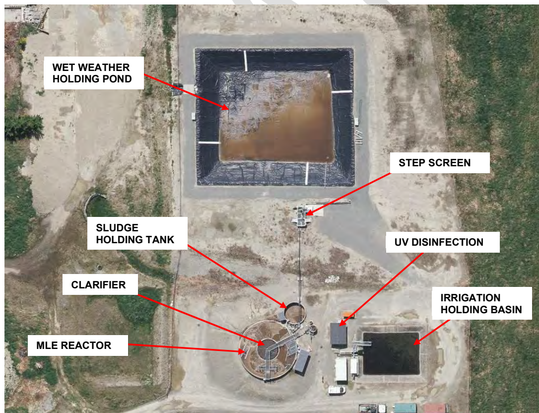
Figure 1 Oxford WWTP aerial view
