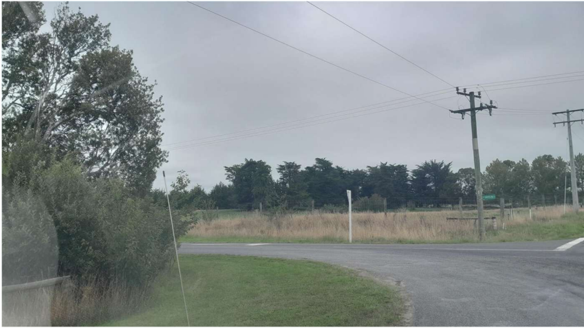
Figure 2: Catherwoods Road / Davis Road intersection with restricted visibility (photo taken from Catherwoods Road looking west towards Davis Road (south approach))
