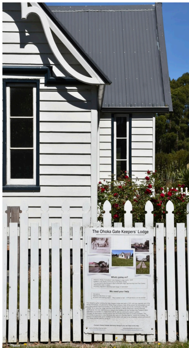
Ohoka Gate Keeper's Lodge
