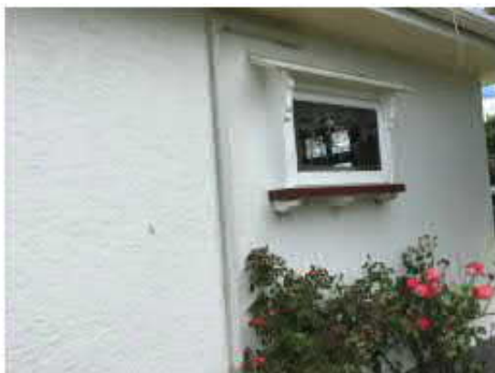
Figure 3: Plastered pre-1940s weather board dwelling.
