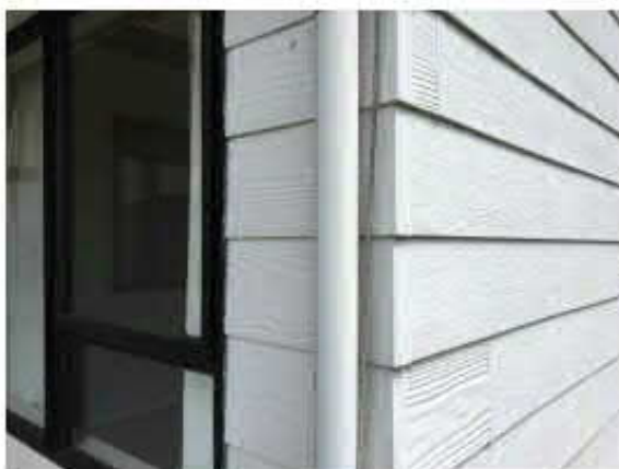
Figure 9: Exterior cladding of the more recent residential dwelling (possibly containing asbestos).
