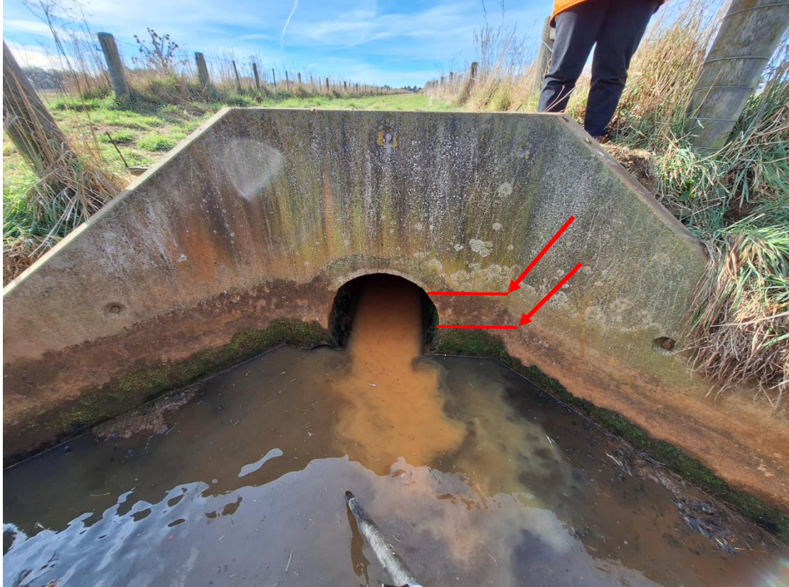
Figure 3: Indication of elevated water levels in the Box Drain pipe network outlet.
