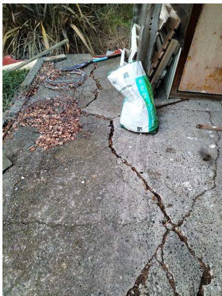
Fig 1.10 a: Cracked Slab on 290 Bradleys Road
