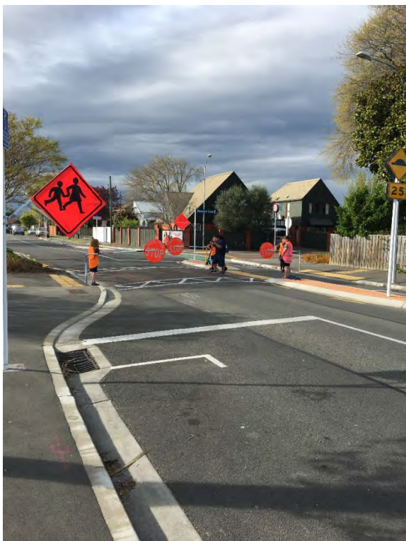
Image 1: Speed management treatment using a raised platform with kea crossing, and road narrowing.
