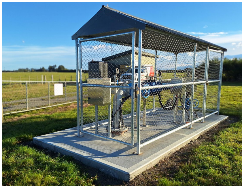
Figure 2. Indicative appearance of wellhead enclosure.
