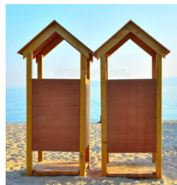
Image 3. Simple standalone change facilities
