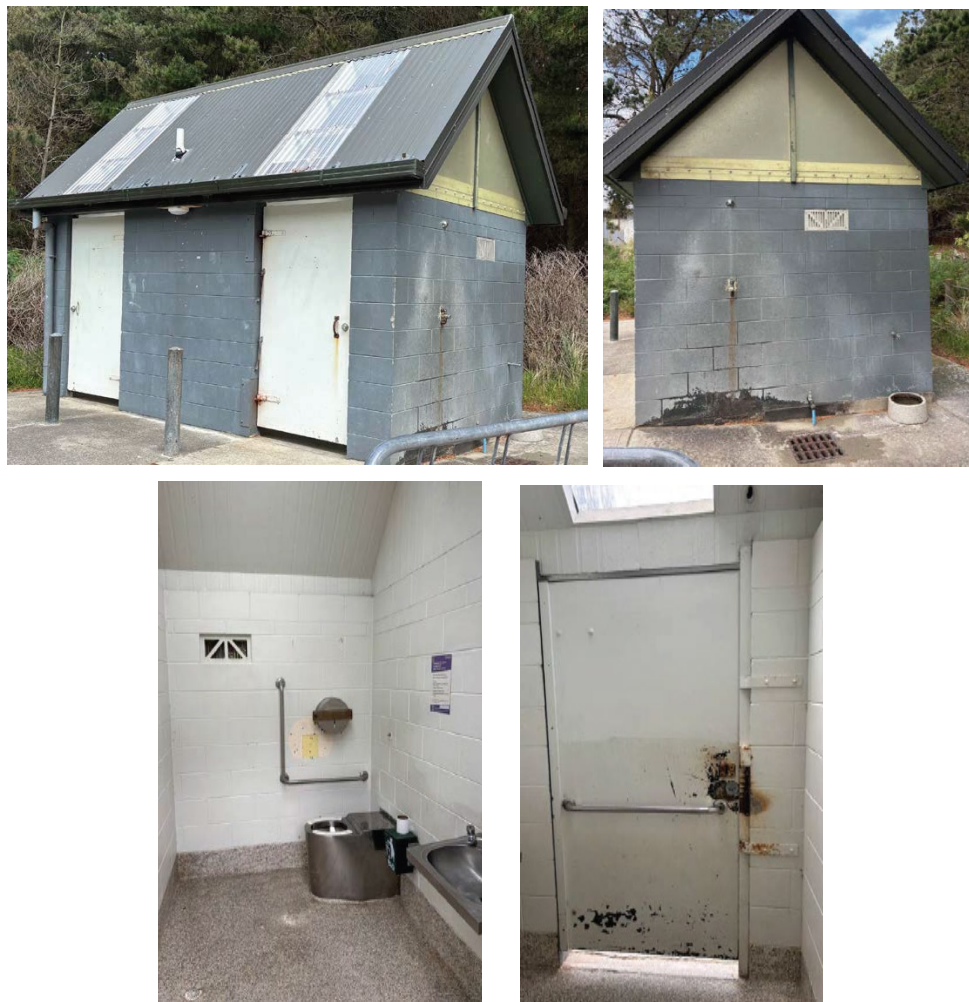
Images 4-7 above: The current exterior and interior state of the Waikuku Beach Toilets
