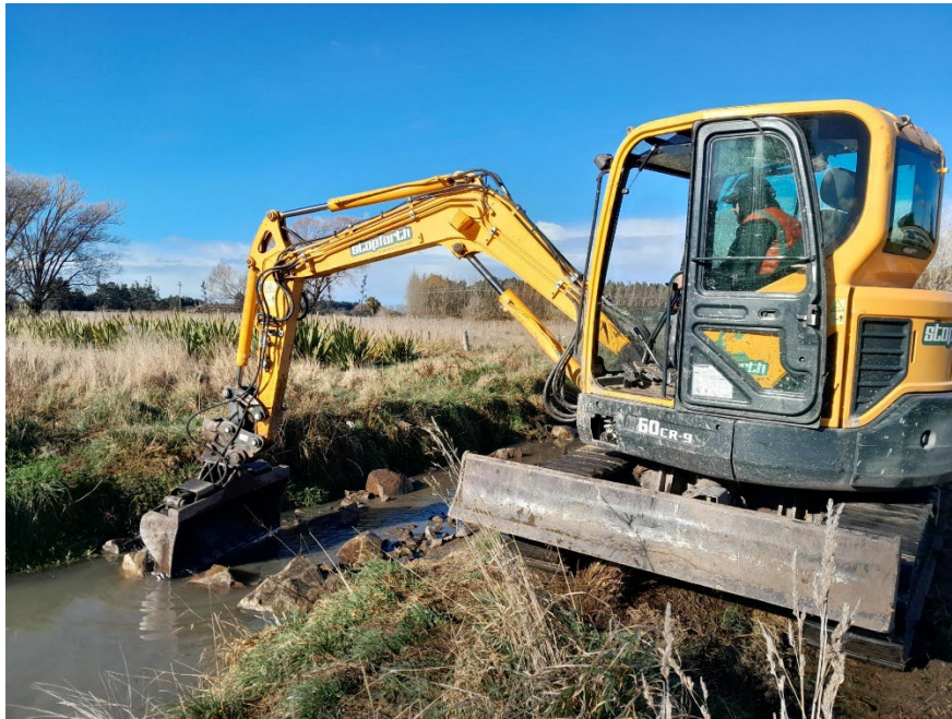
Figure 5: Installation of cobbles and boulders within the Tuahiwi Stream (Waituere) at 428 Tuahiwi Road for aquatic habitat creation.
