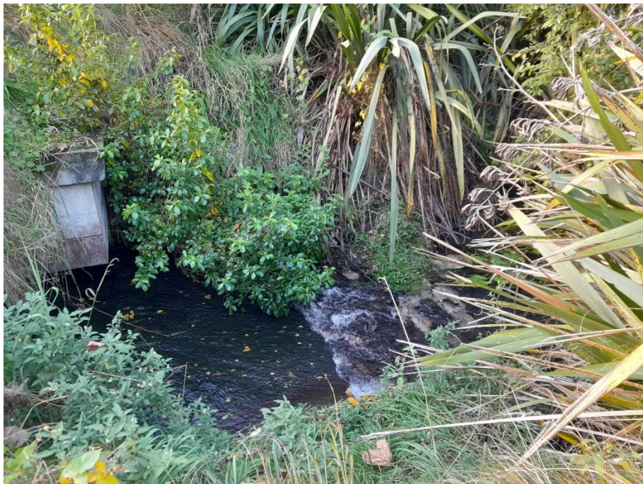
Figure 2: The proposed site of the rock ramp, where a previously installed rock ramp of small cobbles has been scoured away.
