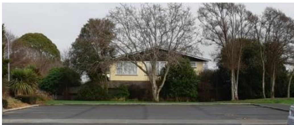
Figure 33: Looking west onto 10 School Road from Woodend Community Centre car park; note the small apparent freeboard between the car park surface and the property boundary
