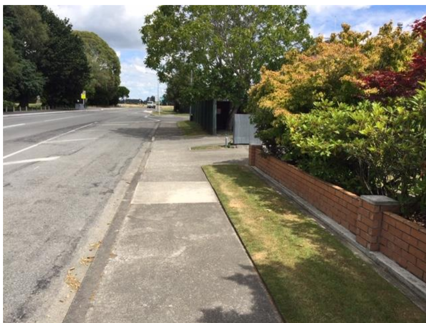
Figure 18: Concrete Brick Wall 10 School Road – Looking Towards Eastern Vehicle Entrance
