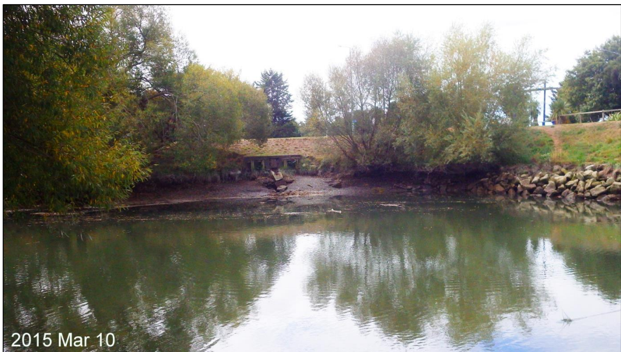
Figure 3.7 Left bank drainage outfall in the elbow bend of the Kaiapoi River
