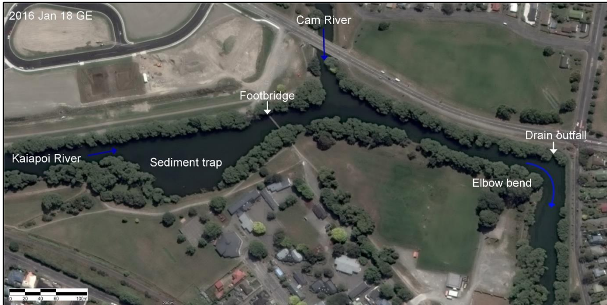
Figure 1.1 Kaiapoi River rehabilitation area Stage 1a – variation reach Jan 2016 (AP Google Earth)
