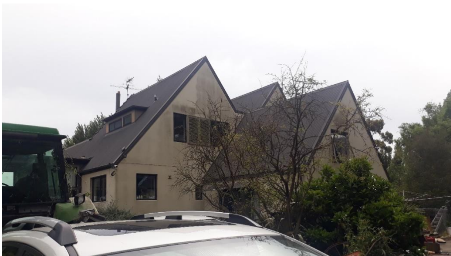
A2 – dwelling at 310 Beach Road - construction materials include suspect ACMs.
