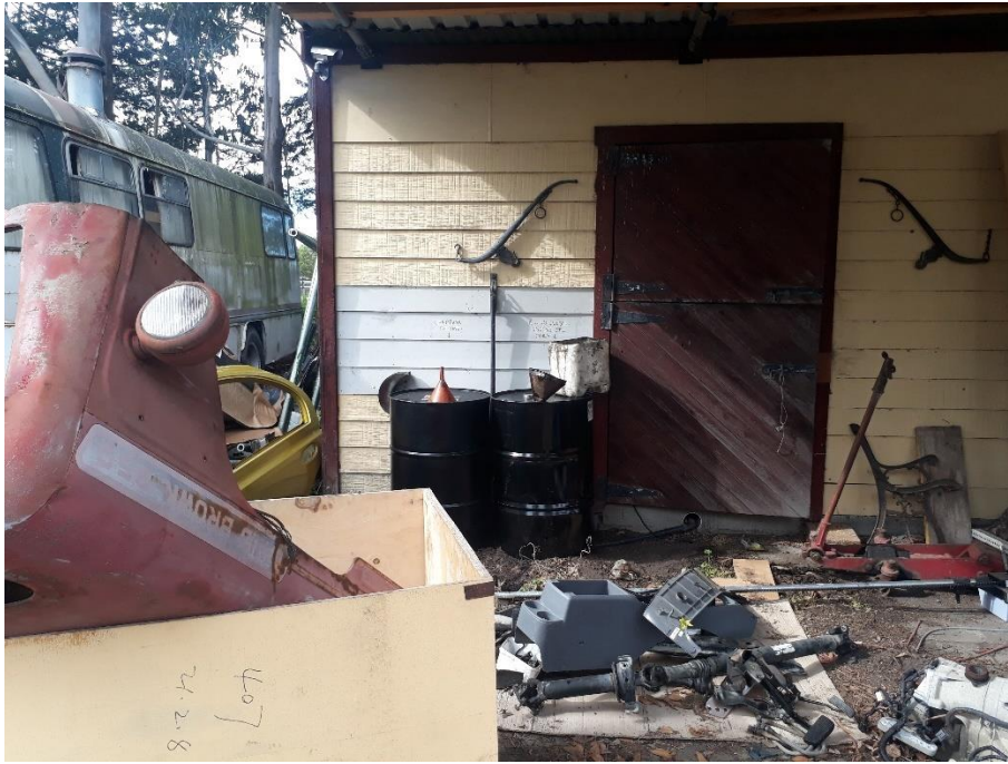
A5 – oil storage at garage outbuilding, Block 1. Note suspect ACM faux wood effect cladding.
