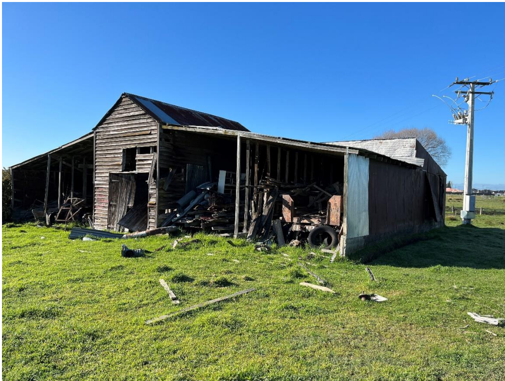
D2 – Barn located in south-western corner of Block 4.
