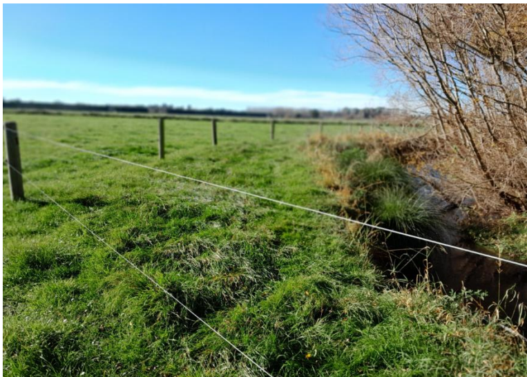
Figure 7: Example of one of the South Brook areas for bank stabilisation.
