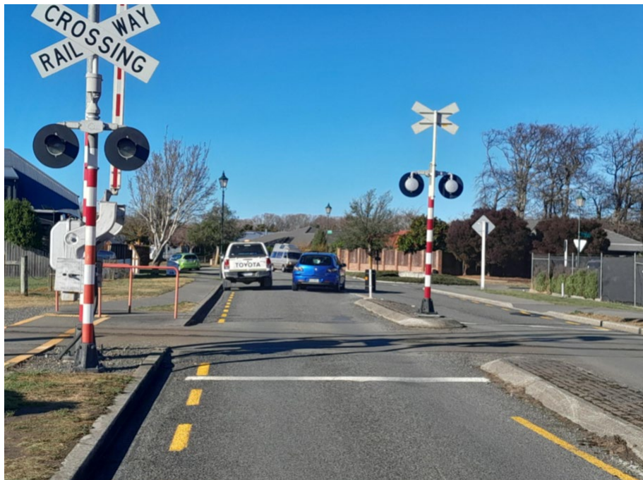
Figure 1 – Vehicles crossing centreline when cars parked at the proposed location.
