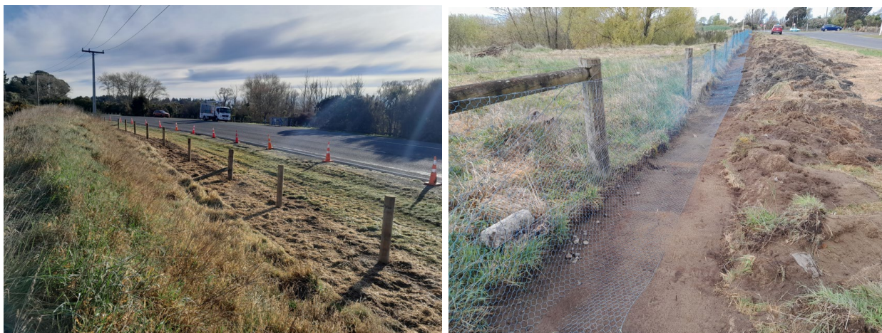
Figure 6. Fence work used the existing posts where possible (left) and covered the netting with rabbit proof fencing as a pest mammal management tool (right).
