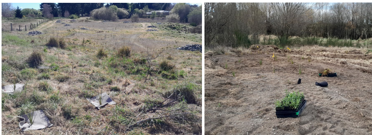
Figure 4. Planting works at Kaiapoi Lakes.
