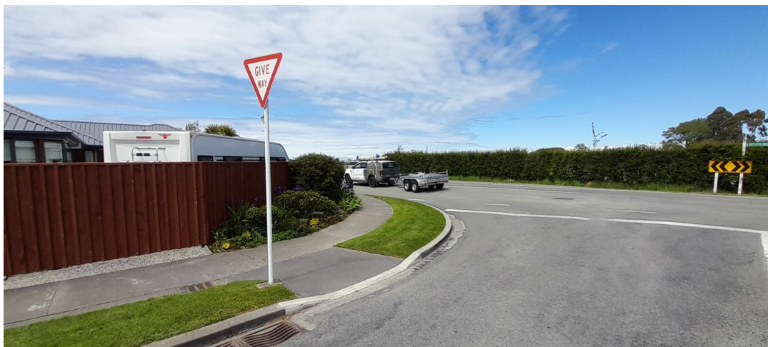
Figure 5: Pentecost Road / South Belt intersection with restricted visibility.
