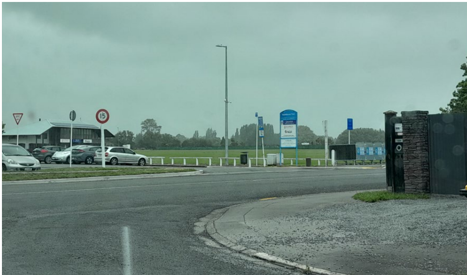
Figure 11: Banks Place / South Belt intersection with restricted visibility.
