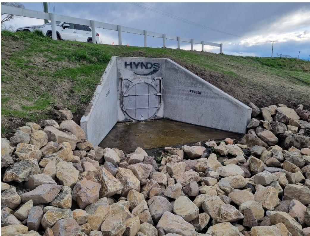
Figure 1 Bradley Road project headwall and flood gate
