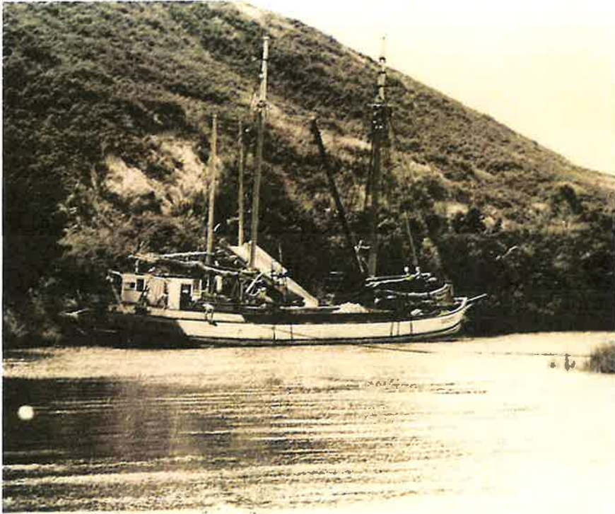
The Scow "Success" loading Fireclay Left bank.
