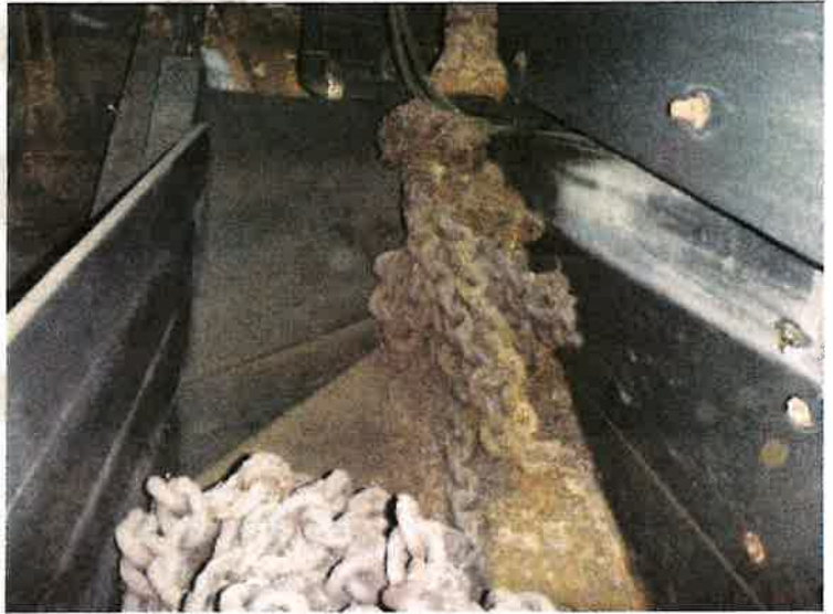
Bow in centre chain locker
