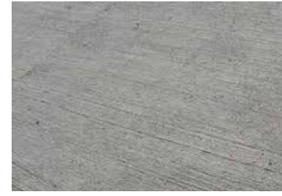
PATHWAYS Broom finish concrete
