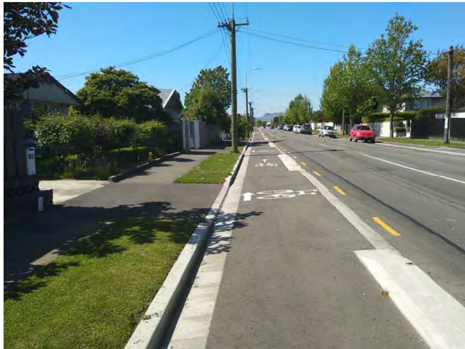
Figure 3. On-road lane with traffic buffer in Christchurch.
