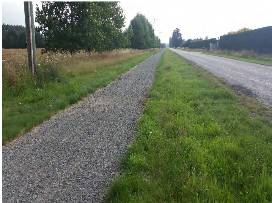
Figure 4. Rural shared path on North Eyre Road.
