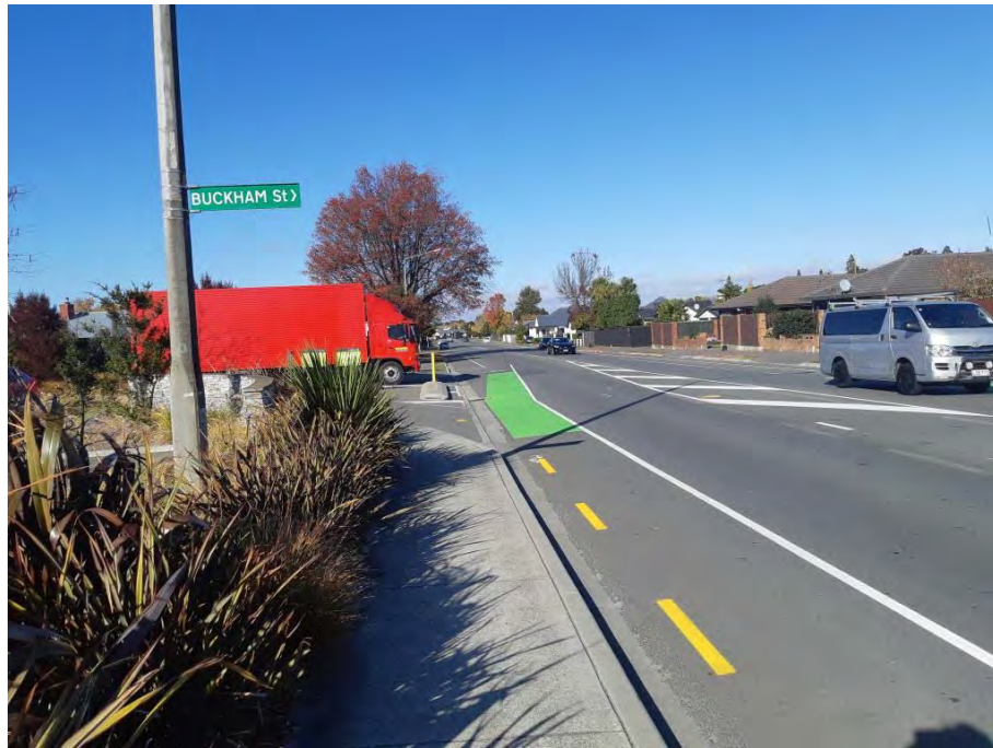
Figure 5. On-road cycle lane on Ivory Street.
