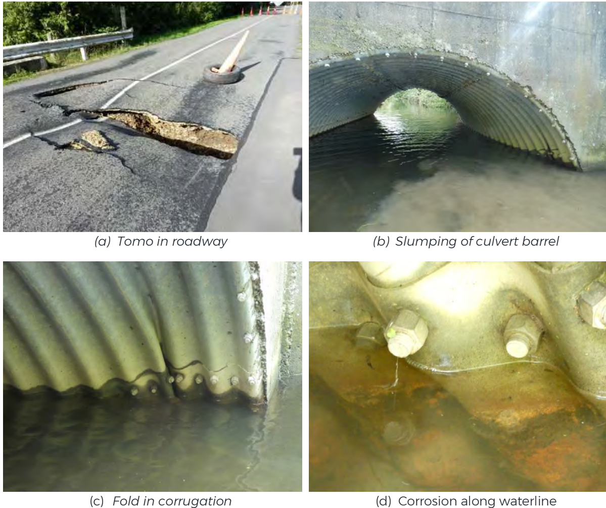
Figure 1-2: Culvert failure
