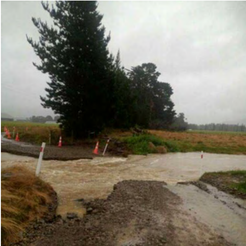
Photo 22 - Taaffes Glen Rd - Reinstated bypass road washed out in Feb event
