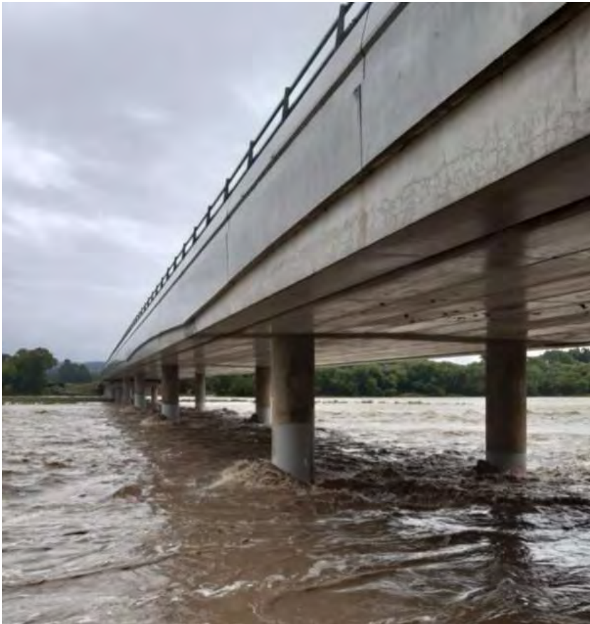
Photo 6 - Ashley River Bridge
