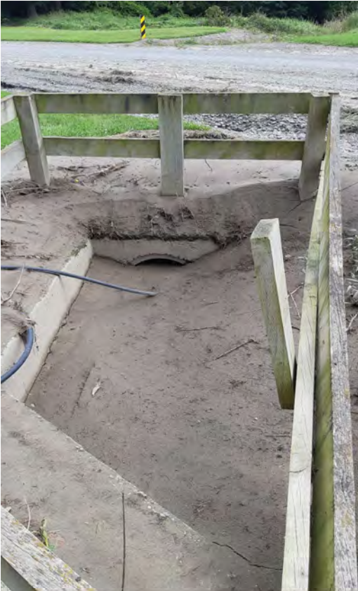
Photos 20 & 21 - Heyland Rd blocked culvert and road scour
