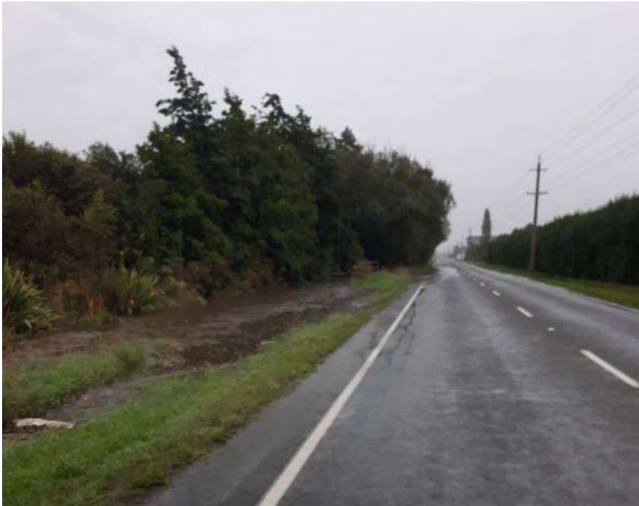
Photo 7 - Flaxton Rd east of Fernside Rd – Surface flooding onto road
