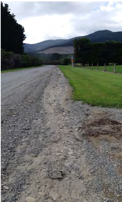
Photos 20 & 21 - Heyland Rd blocked culvert and road scour
