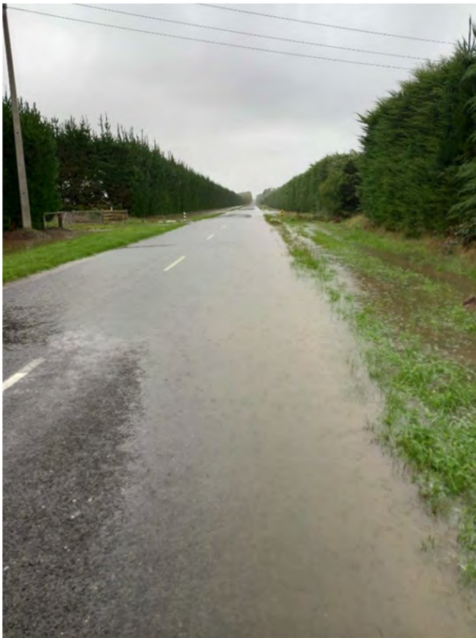
Photo 8 - Poyntz Rd Surface Flooding
