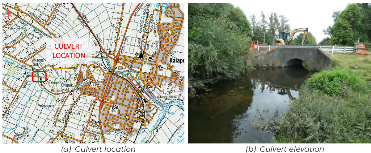
Figure 1-1: Butchers Road Culvert
