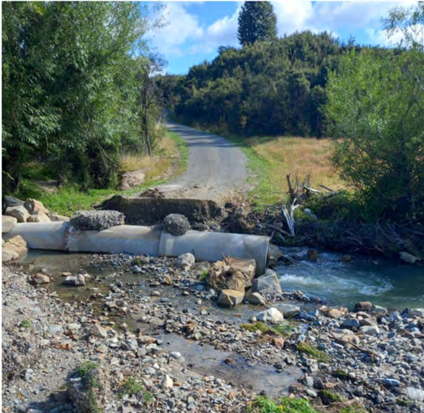
Photo 10 - Okuku Pass Rd - Culvert Scour Repair
