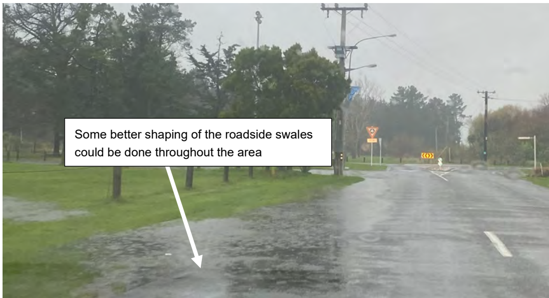
Figure 9: Dunns Ave looking toward roundabout (1 May 2025).
