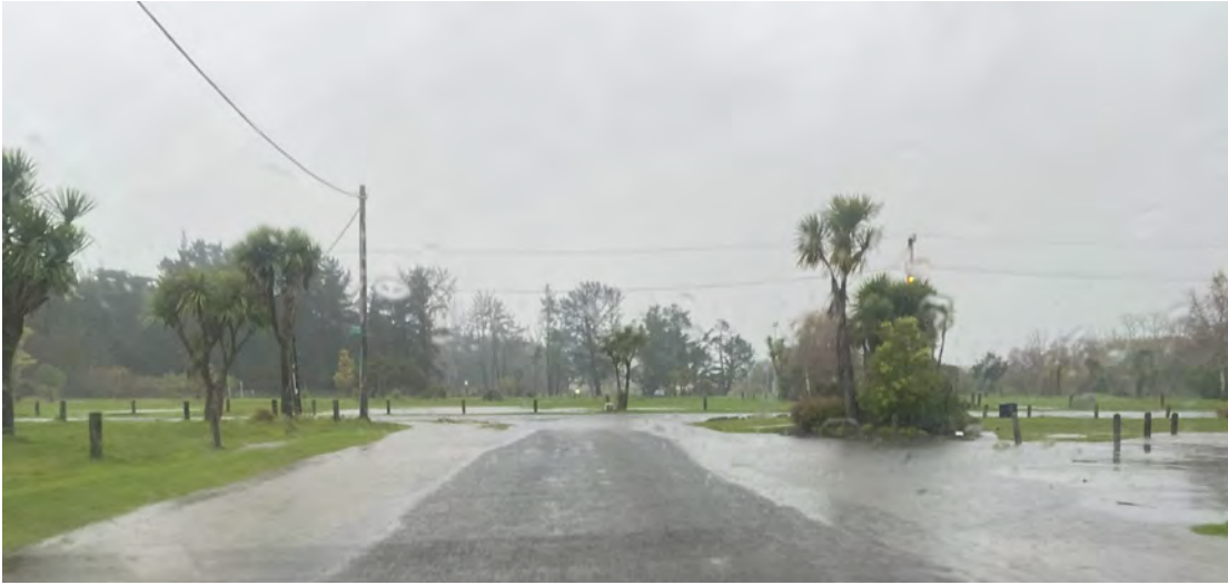
Figure 3: Example of roadside swale flooding. Southern end of Batten Grove (outside Pines Beach Hall) (1 May 2025).
