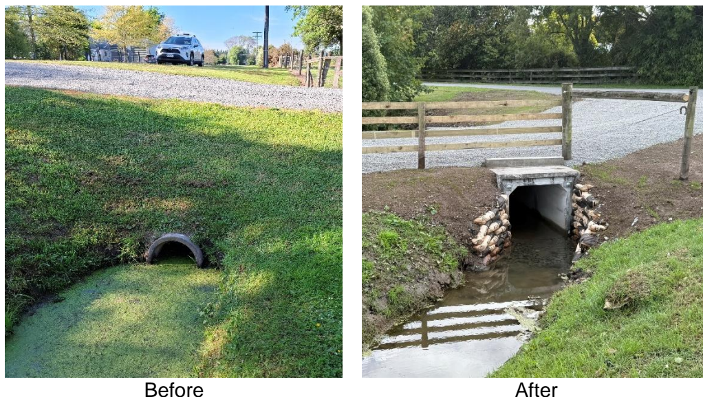
Figure 2 Before and after construction of the box culvert
