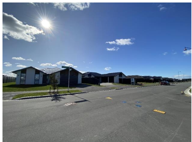
Figure 6 - Completed Houses in Beach Grove Subdivision - Kaiapoi
