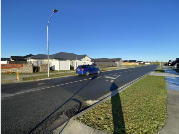
Figure 1 - Houses Already Constructed in Townsend Fields Rangiora
