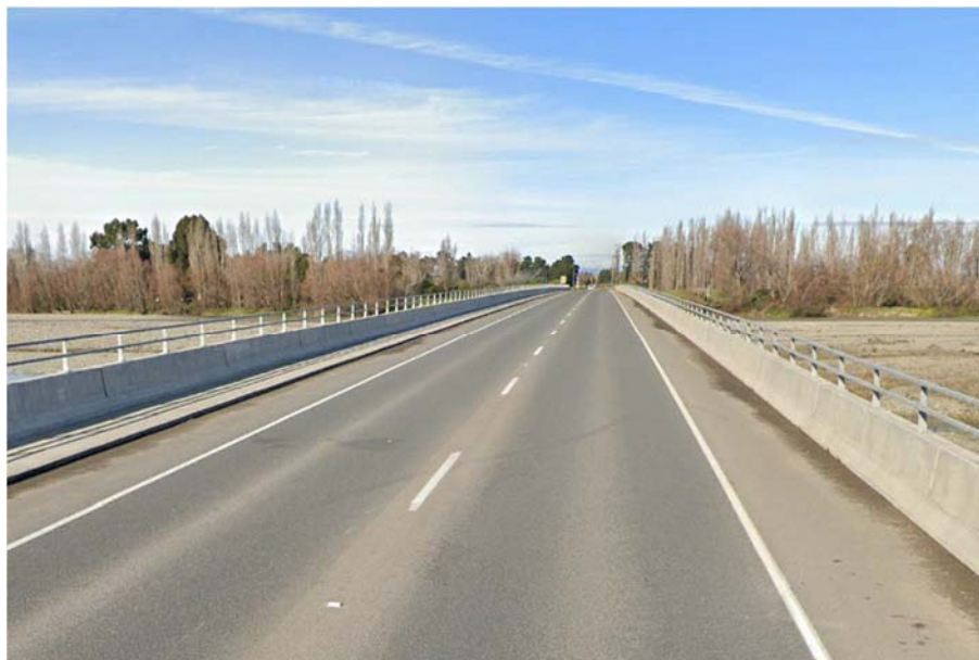
Photograph 6: Wide Shoulders and Separated Footpath on Ashley Bridge (Looking South)
