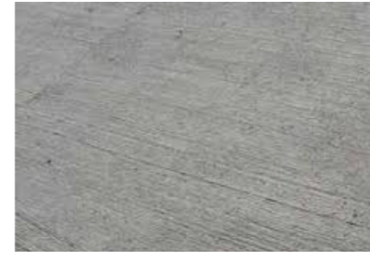
PATHWAYS Broom finish concrete
