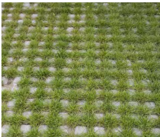
Figure 3. Example of reinforced shoulder product (Firth Gobi® Block).
