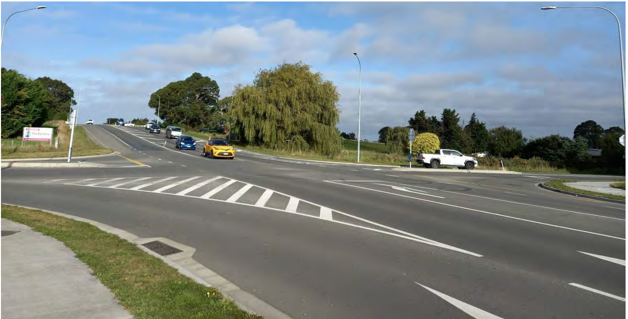
Figure 4 Current Ohoka Road/Island Road intersection – view for the southwest corner
