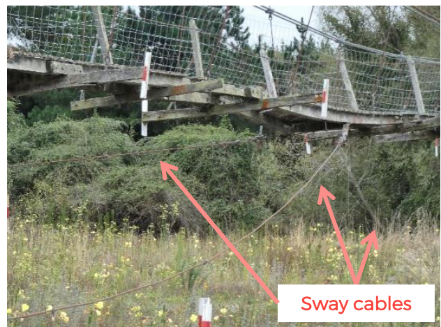
Figure 3.14: West abutment sway cables
