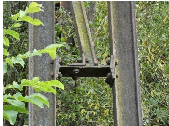
Figure 5.2: Tower steel member condition – western tower
