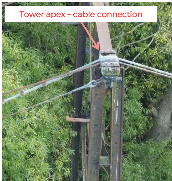
Figure 3.7: Cable tower connection - west abutment - downstream side
