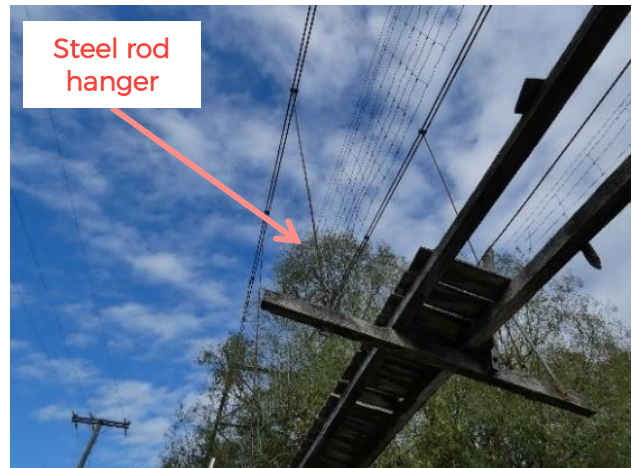
Figure 2.2: Typical steel rod hanger
