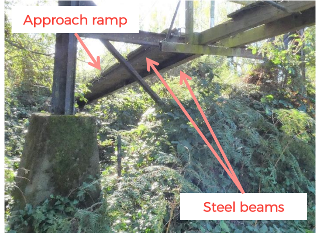
Figure 1.11: East approach ramp - underside
