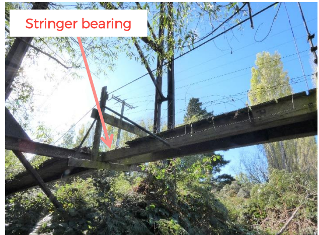
Figure 1.2: East abutment stringer bearing
