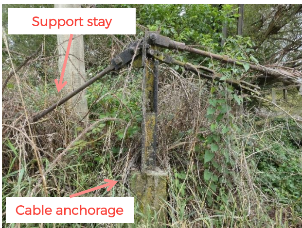
Figure 4.5.3: Western downstream sway cable anchorage
