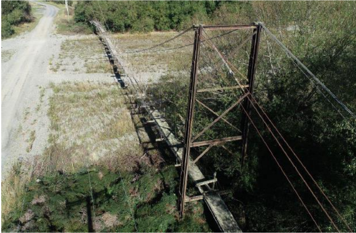
Wolffs Road suspension bridge – West Eyreton
