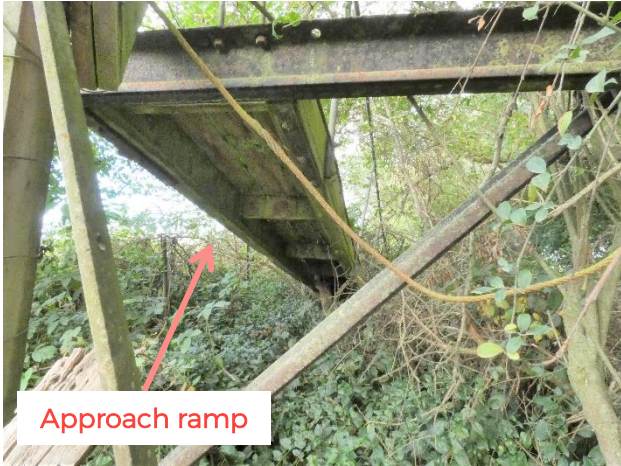
Figure 1.10: West approach ramp - underside
