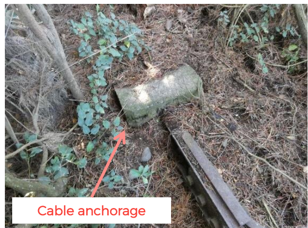
Figure 4.4: Eastern upstream cable anchorage block
