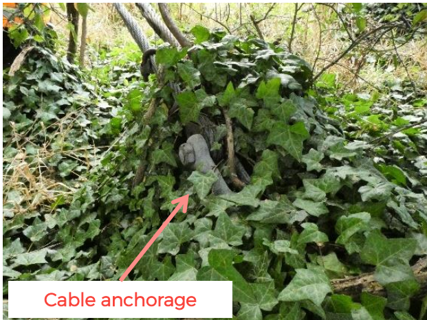
Figure 4.5.1: Western downstream cable anchorage - unable to be visually inspected
