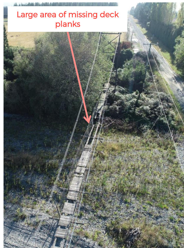
Figure 4.1.2: Deck plank condition overview – facing east abutment
