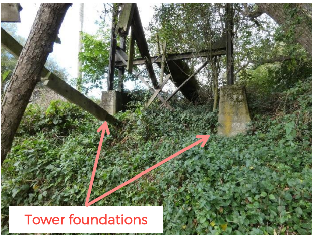
Figure 4.6.2: Tower foundations - western tower
