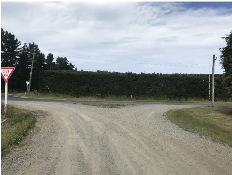
Photograph 2-4: Priors Road/Merton Road intersection west approach
