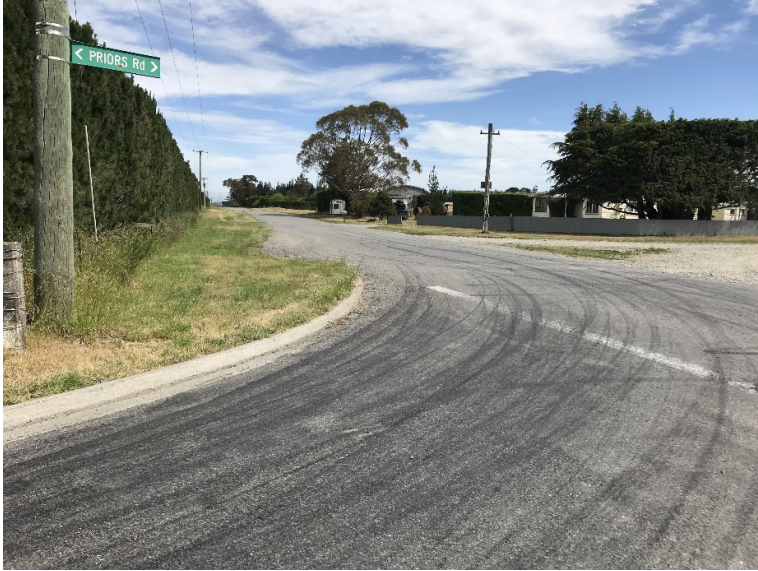
Photograph 2-3: Priors Road/Merton Road intersection looking south
