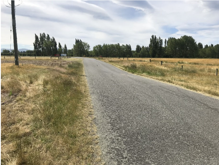
Photograph 2-1: Merton Road north of Priors Road intersection
