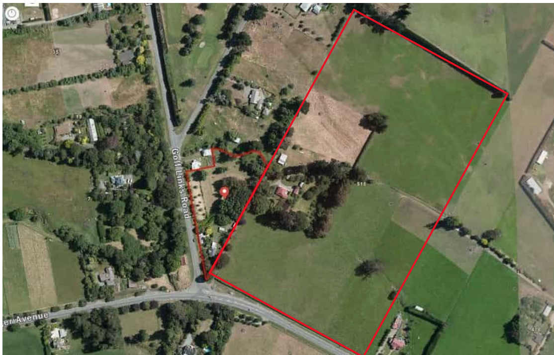
Aerial imagery of 4 Golf Links Road (left) and 518 Rangiora Woodend Road (right) between 2010- 2014 (site boundary outlined in red). Retrieved from Canterbury Maps.
