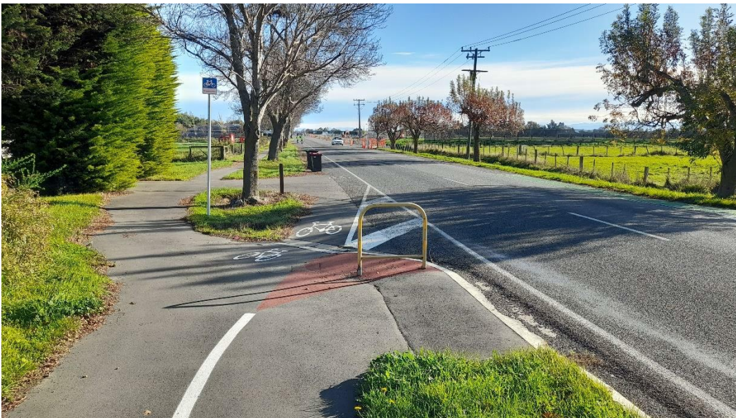
Photograph 3-15: Off-Road Path Transition to On-Road Cycle Lanes
