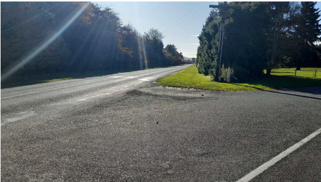
Photograph 3-11: Marchmont Road Sightline to Right at Golf Links Road
