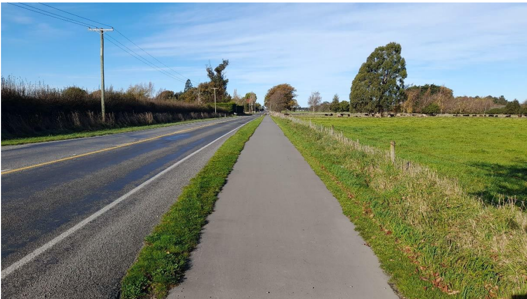
Photograph 3-13: Rangiora Woodend Path, Looking East
