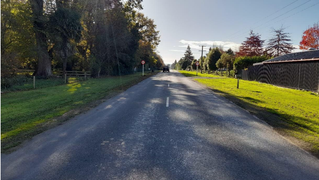
Photograph 3-5: Golf Links Road Looking North (Site on Right)
