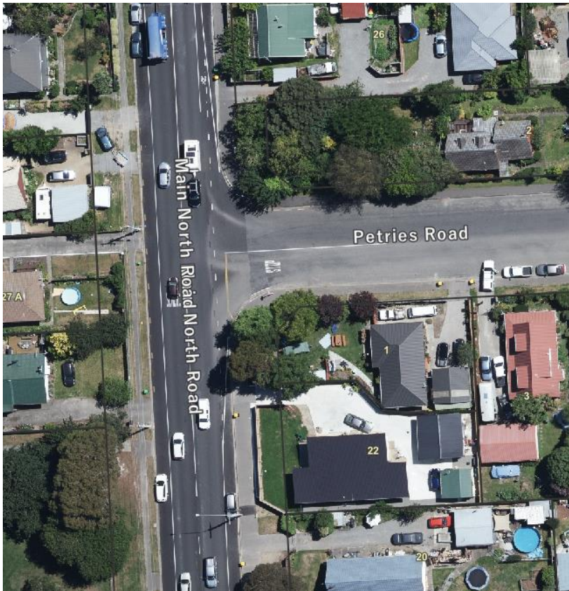
Figure 3.2 Intersection of Main North and Petries Roads. (Source: Canterbury Maps).
