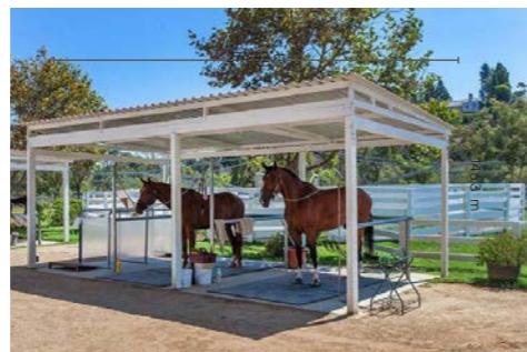
Bespoke facilities will be provided
