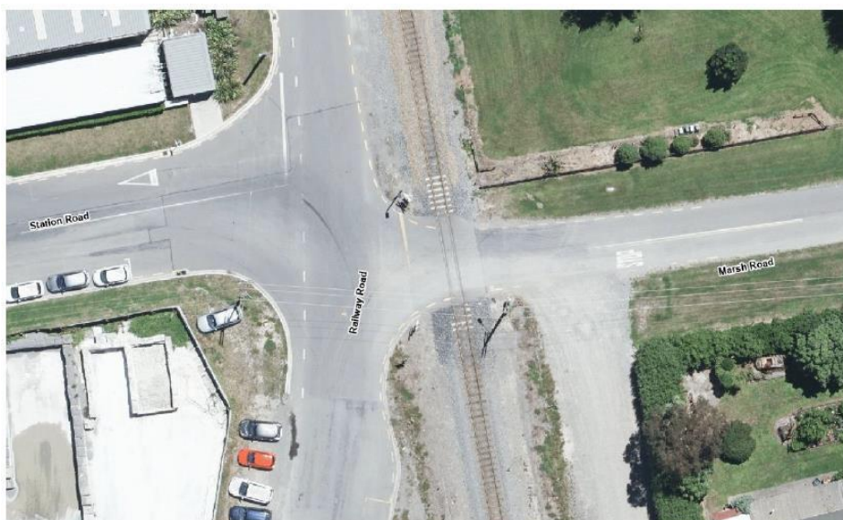
Figure 4-2: Marsh Road level crossing aerial (Canterbury Map Viewer)
