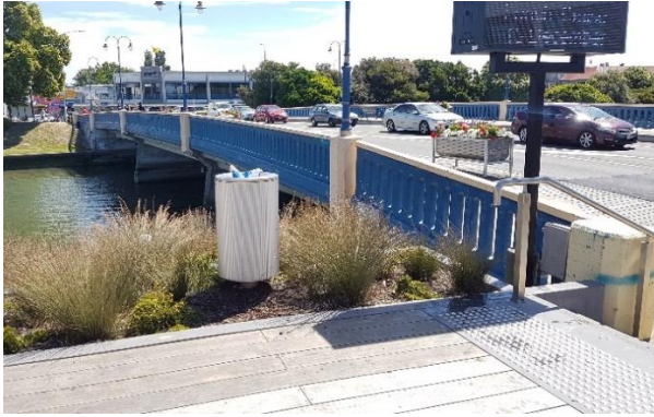
Figure 2-3: View from north
