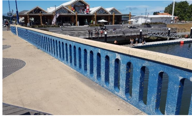
Figure 2-4: View from bridge
