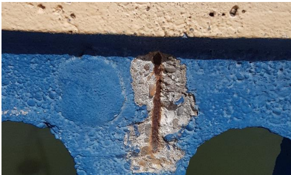
Figure 2-5: Spalling
