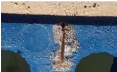
Figure 5 – Spalling
