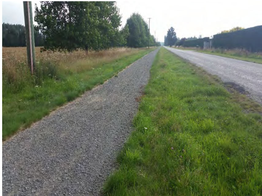
Figure 4. Rural shared path on North Eyre Road.
