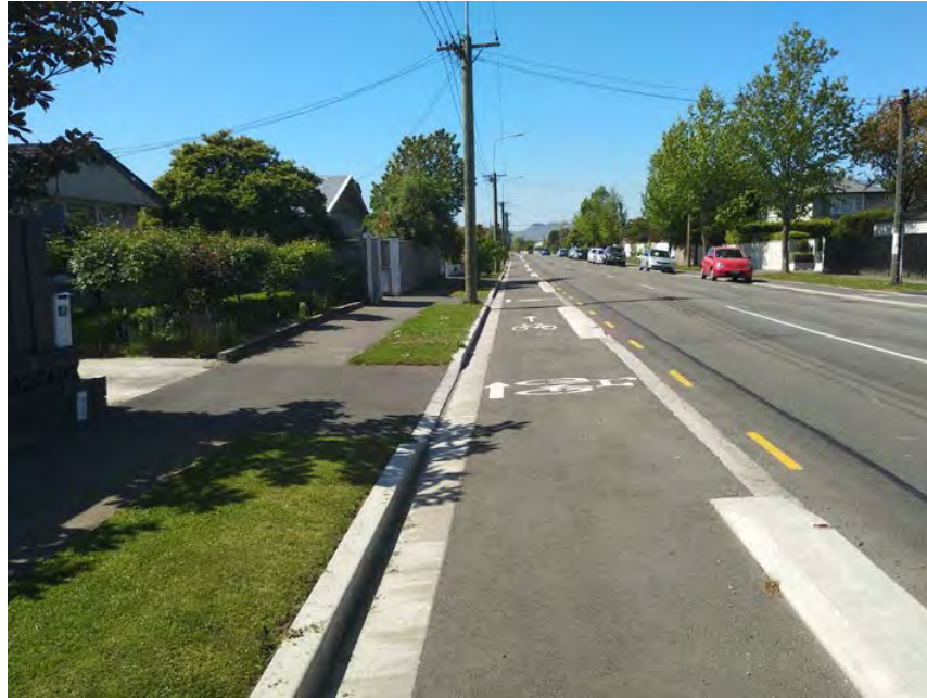
Figure 3. On-road lane with traffic buffer in Christchurch.
