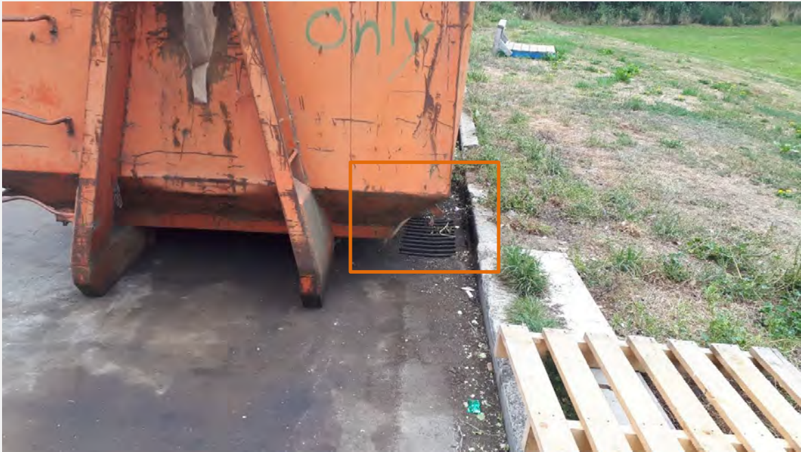
Figure 4: Stormwater sump at risk of receiving contaminated stormwater.
