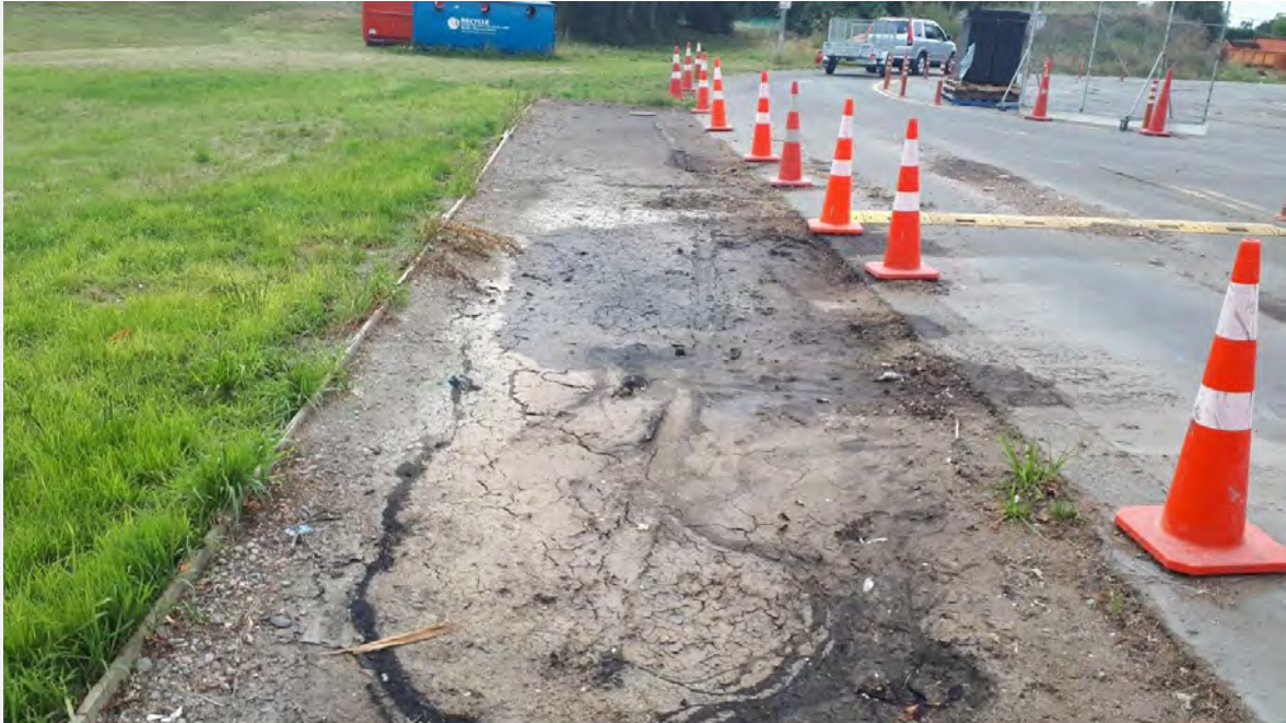
Figure 5: Recently constructed stormwater pad.
