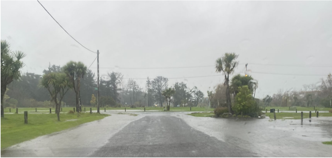
Figure 3: Example of roadside swale flooding. Southern end of Batten Grove (outside Pines Beach Hall) (1 May 2025).
