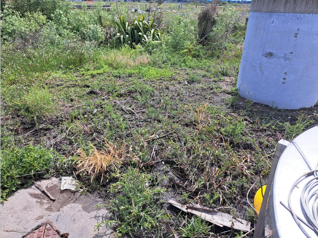
Figure 4: Standing on the eastern wet well looking north to the South Brook with dark coloured grass from the sewage overflow
