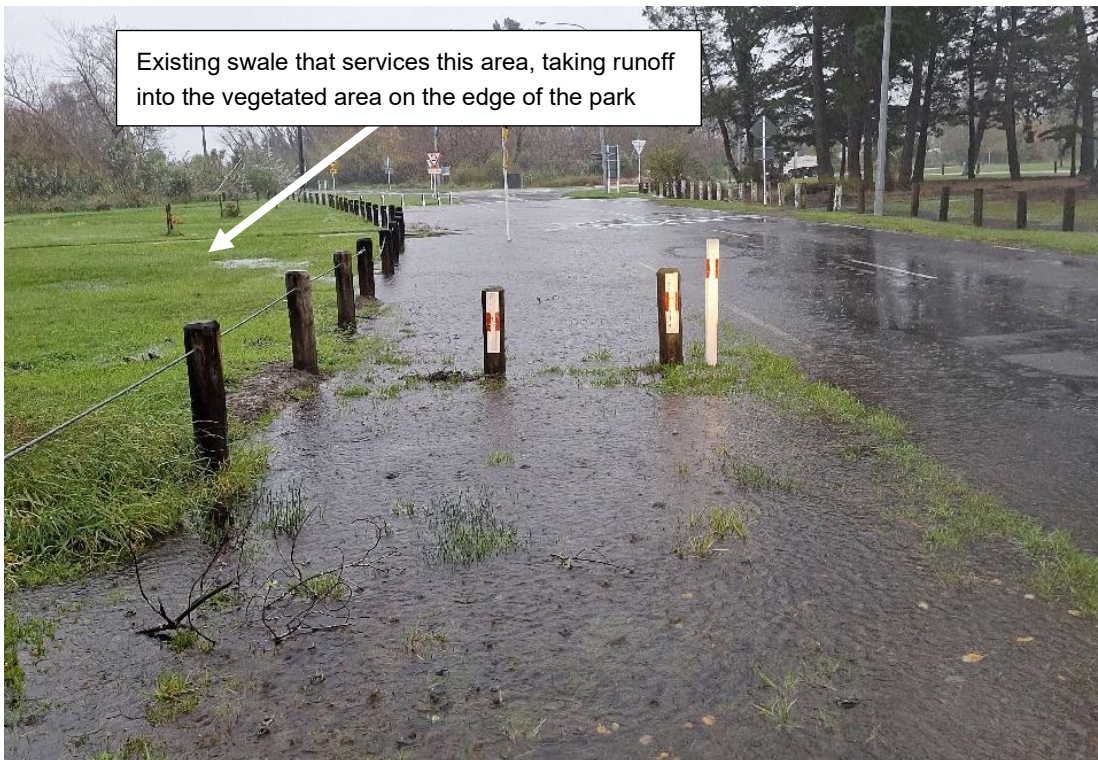
Figure 10: Featherstone Ave looking north to the roundabout (1 May 2025).
