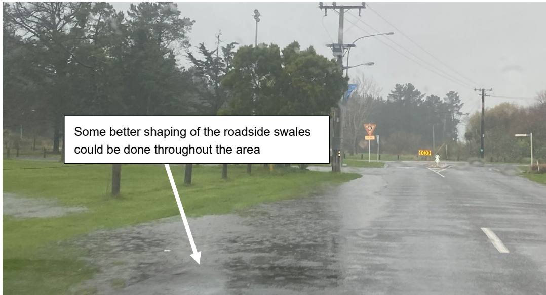
Figure 9: Dunns Ave looking toward roundabout (1 May 2025).
