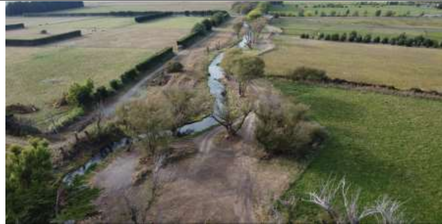
Cam River Maintenance Works
