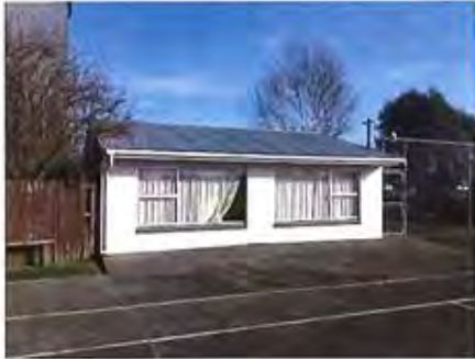
Clubrooms exterior (court face)
