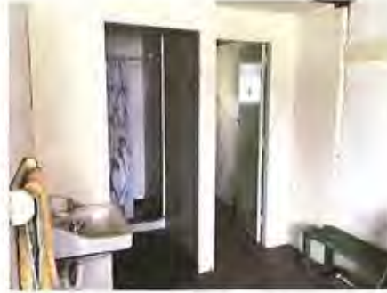
Ground floor changing room and ablutions
