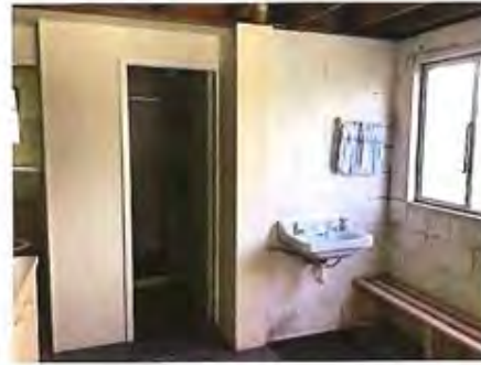
Ground floor changing room and ablutions
