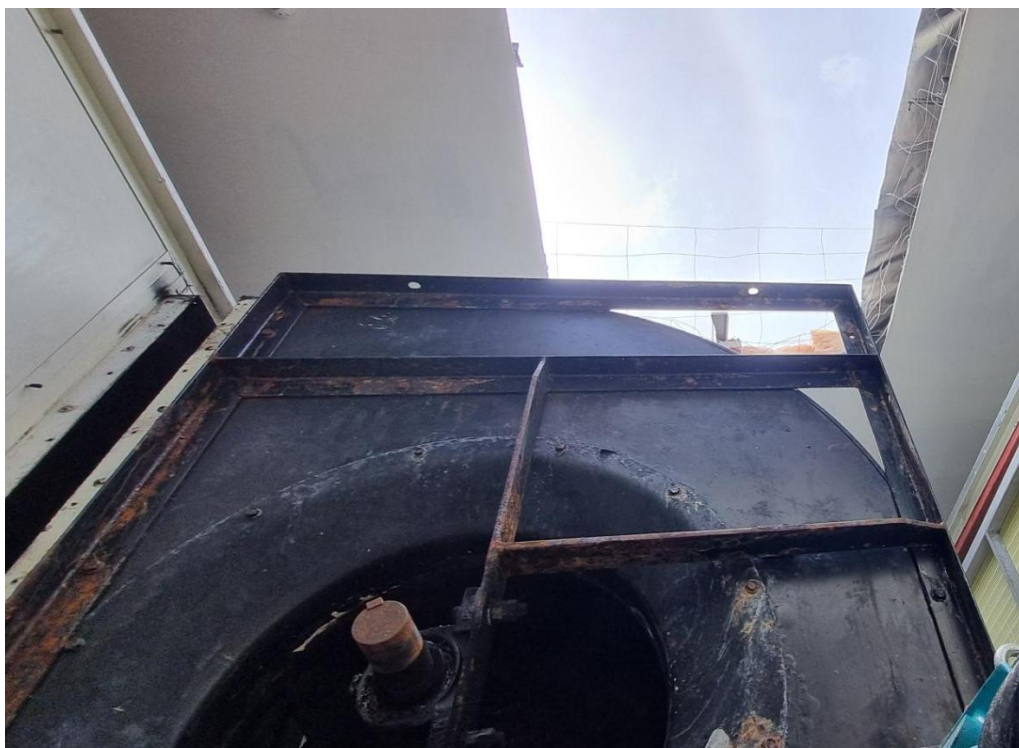
Pictured: The old fan showing signs of wear and tear and the hole in the ceiling it was removed through.
