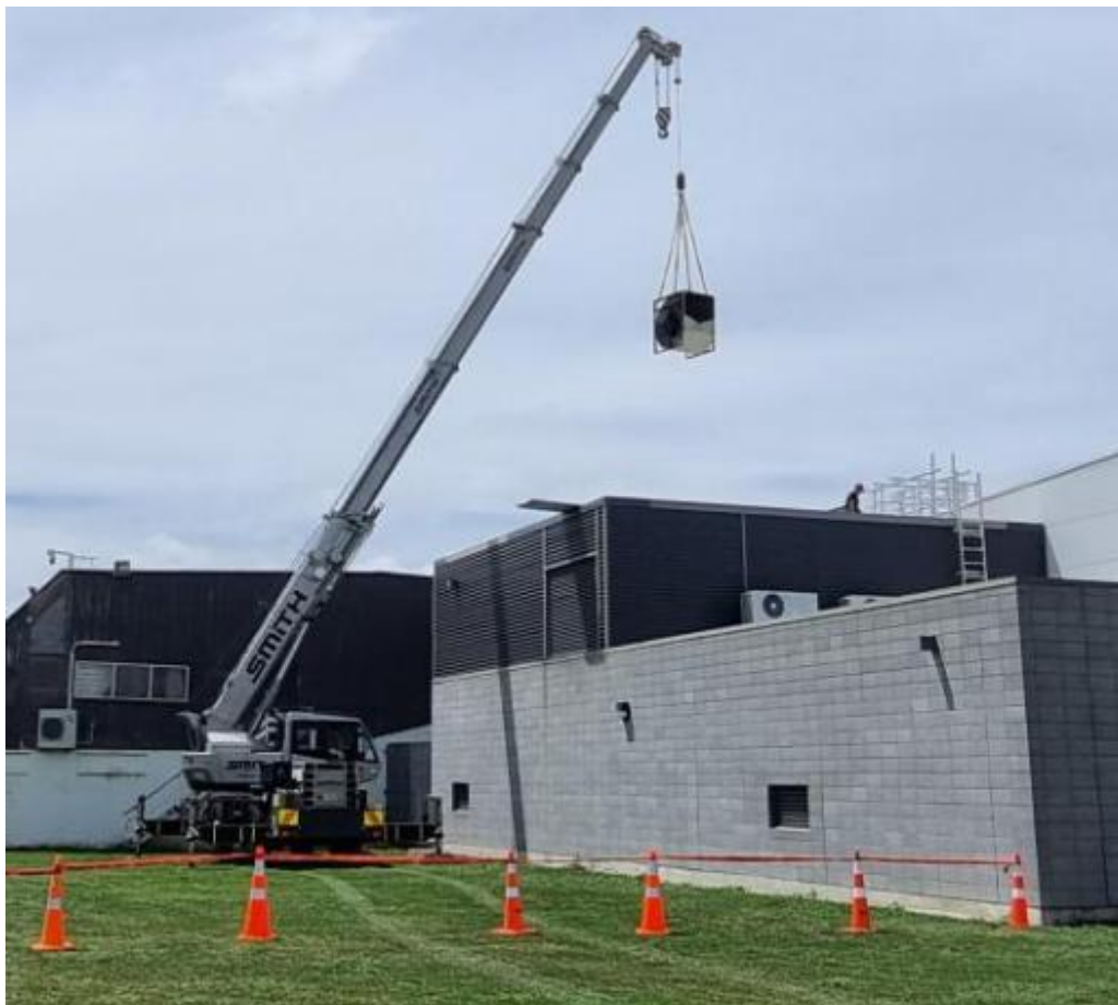
Pictured: A crane is used to remove the old fan through a hole in the ceiling of the plant room.
