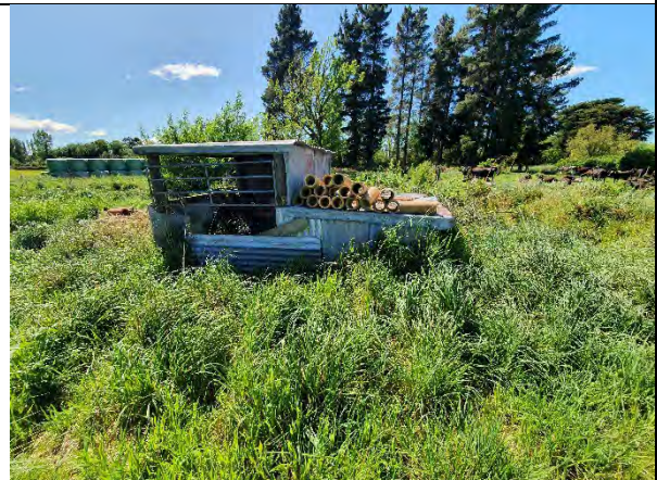
P34: Small shed located along northern perimeter of Block A which is generally used to store lengths of clay pipe.
