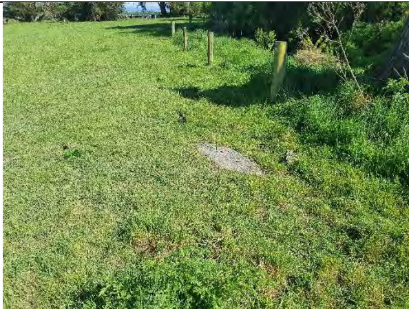
P3: Evidence of buried concrete in infilled area.
