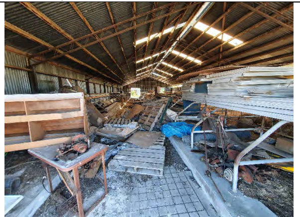
P28: Internal view of large shed.
