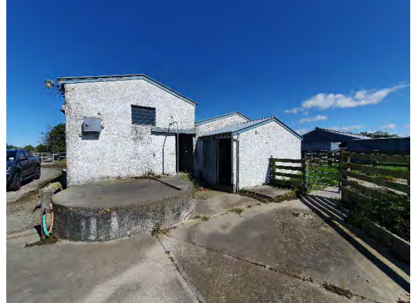
P16: Close up of milking sheds, which appear to be clad with some type of stucco type cladding.
