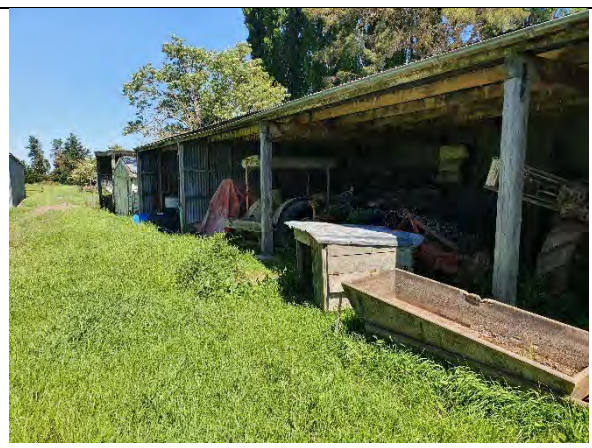
P51: Lean to implement shed with earthen floor along eastern side of large shed. Used to store various old farm equipment.
