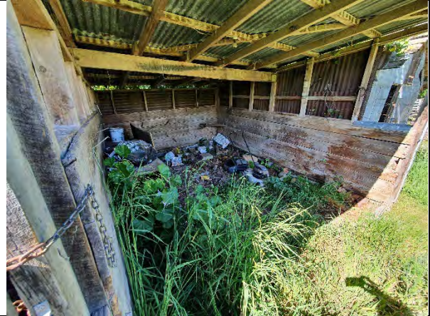
P8: Internal view of sheds.
