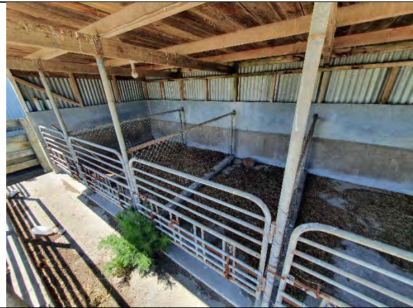
P22: Internal view of shed, showing concrete floor.
