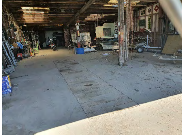
P46: Western half of large shed. The feature on the floor looks similar to a vehicle inspection pit indicating possible historical use as a workshop.
