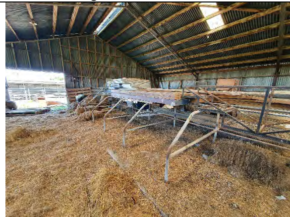
P29: Internal view of large shed.
