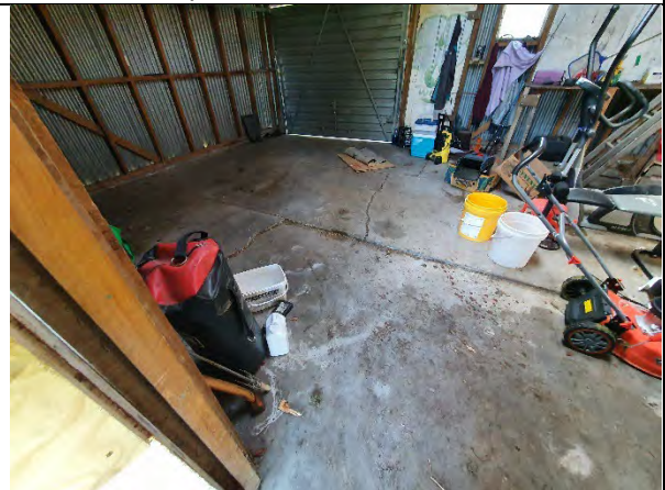
P12: Internal view of garage.
