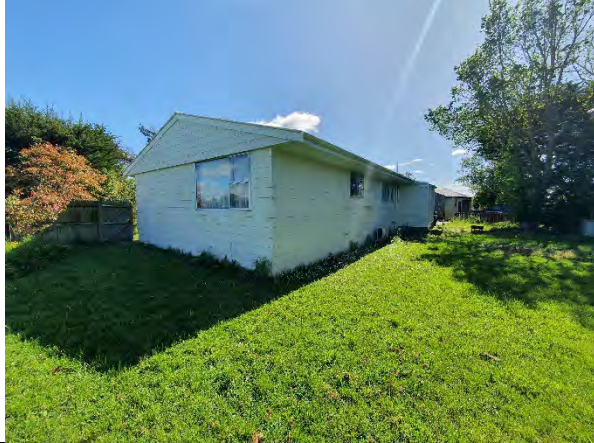
P13: Dwelling located in eastern corner of Block A (162 Boys Road). This dwelling is inferred to be a replacement for a previous dwelling burnt down in the early 1980s.
