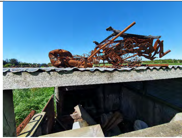
P33: Close up of items (old drums and machinery) on top of shed which appear to have been subjected to heat (i.e. possibly burnt in burn pile).
