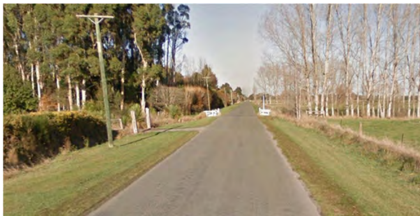
Figure 2: Whites Road Looking South
