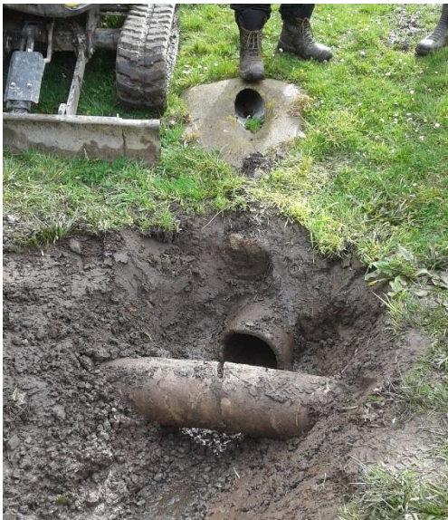
Figure 2. Reserve Road water main and drainage outlet to lagoon.
