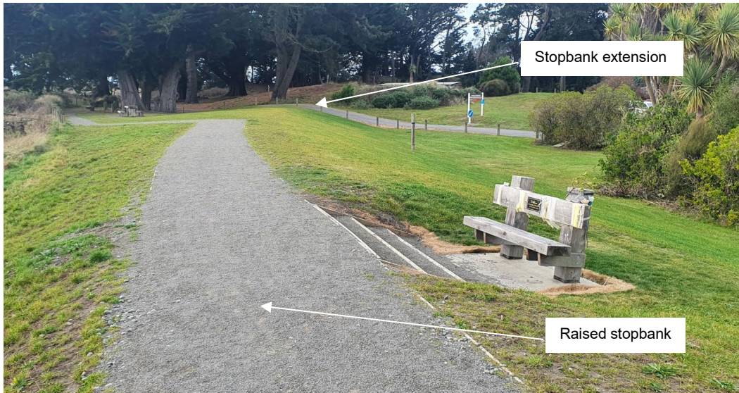
Figure 2 – Photograph of modified stopbank at the Ashley-Rakahuri River Mouth reserve entrance
