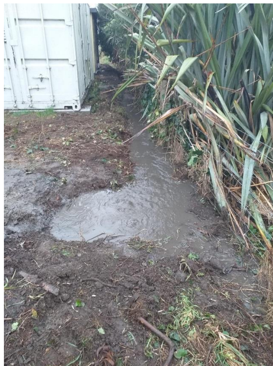
Figure 7. Kings Avenue downstream bubble-up sump opposite 37 / 39 Kings Avenue, and drainage path to the north behind the water pump station.
