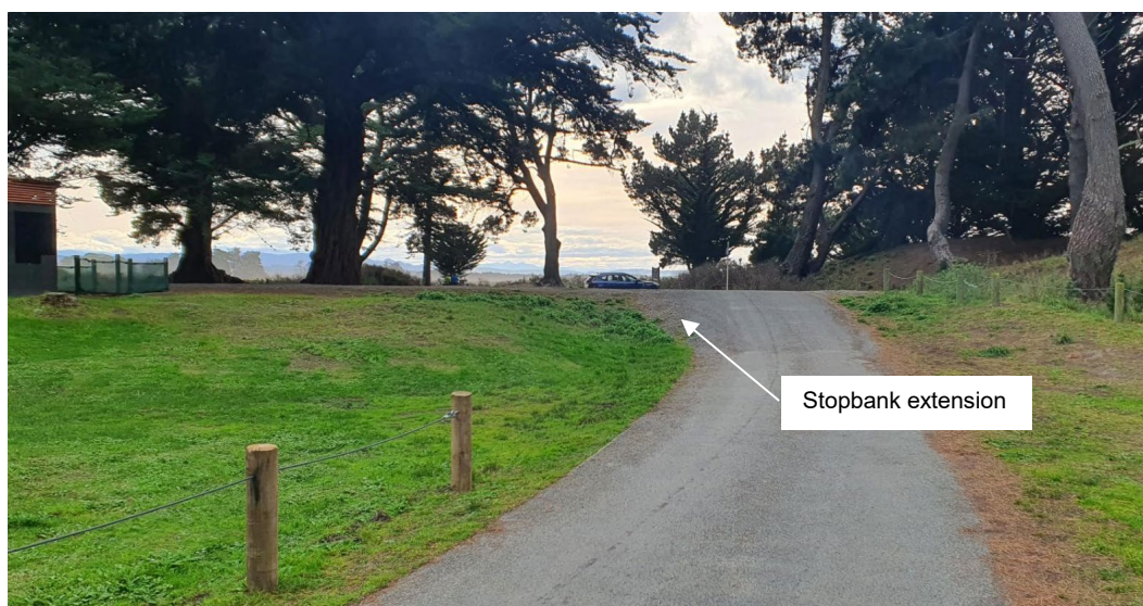
Figure 1 – Photograph of stopbank extension where flow occurred in the May 2021 event
