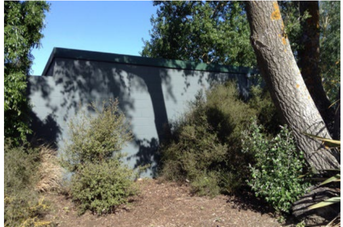
Toilets at the Ashley Picnic Ground are partially obscured by vegetation
