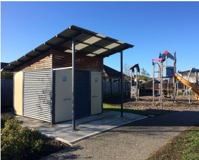
Standard toilet at Bayliss Drive Park, Kaiapoi
