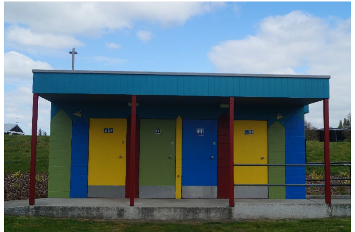
Multi cubicle toilet block at Tom Ayers Reserve with 'friendly appearance' and doors opening straight onto the reserve
