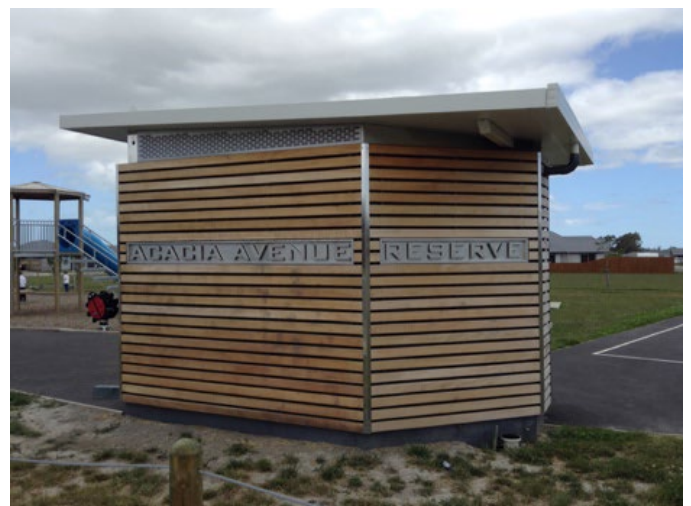
New toilet facilities at Acacia Avenue Reserve, Rangiora
