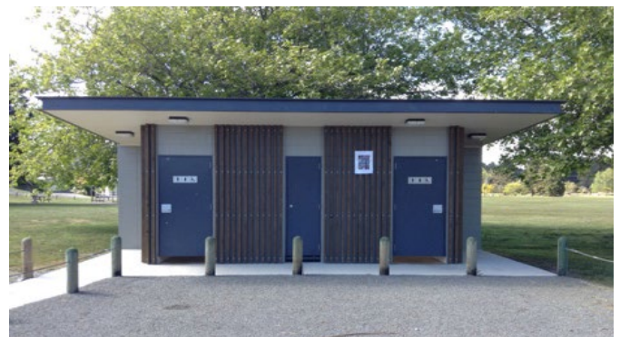
High quality bespoke toilet at Pines Oval, Pines Beach
