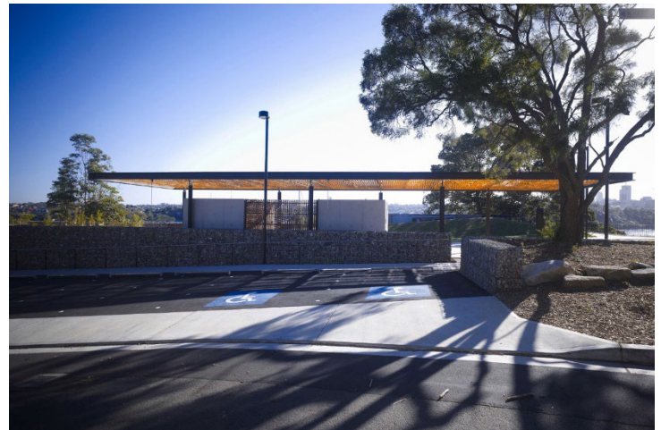
Modern public toilets in Ballast Point Park, Australia
