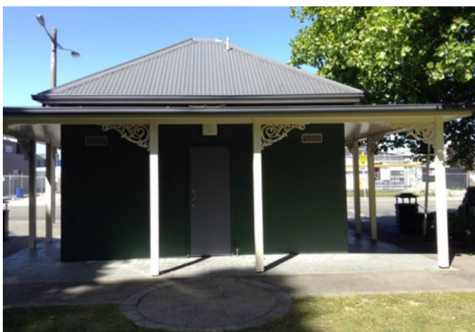
Public toilet at Victoria Park, Rangiora
