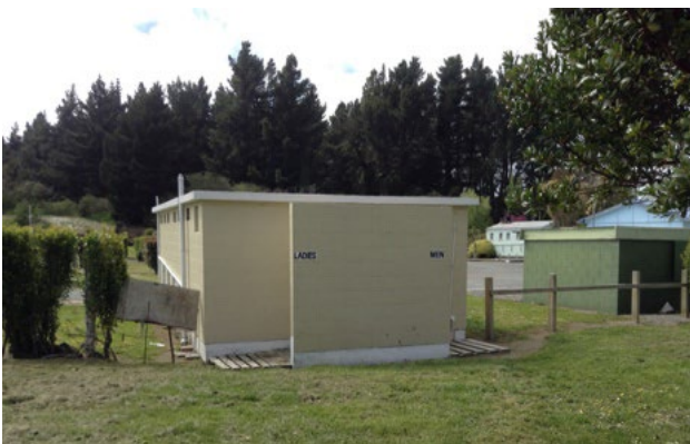
Toilet block on Kairaki Reserve at Kairaki Beach
