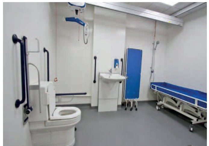
Toilets illustrating good practice inclusive access, large internal circulation space, and inclusive fittings and fixtures
