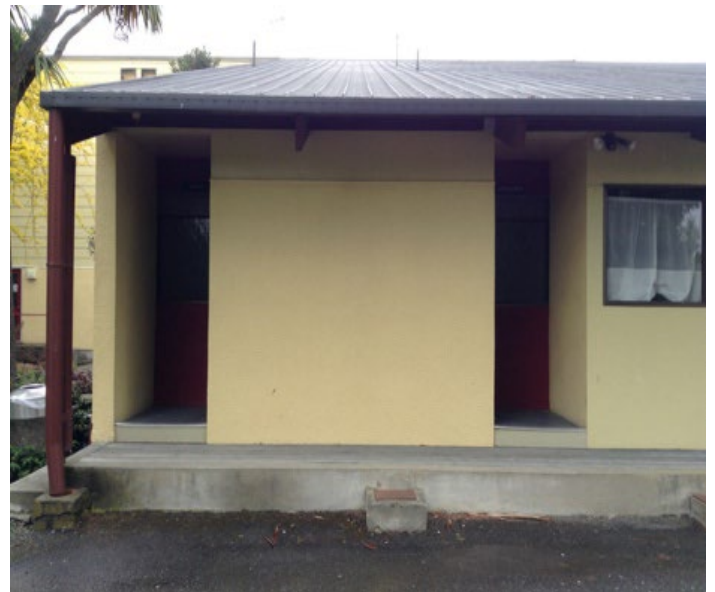
Public toilet at Cust Community Centre – neighbourhood park (community)
