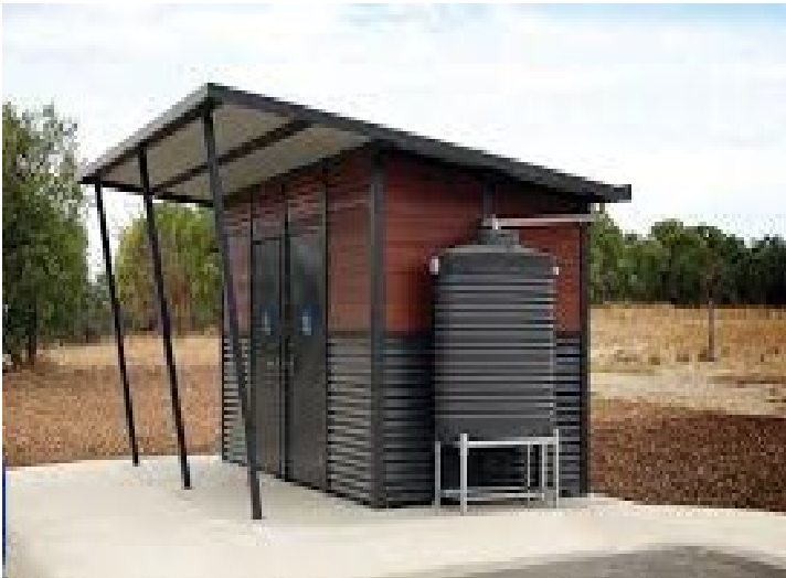
Kitset public toilet in Australia with roof water rain collection tank
