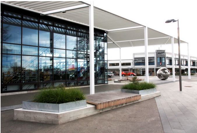
Town centre toilets in the Ruataniwha Kaiapoi Civic Centre
