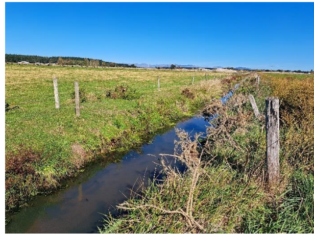
Photo 15: McIntosh Drain looking downstream
