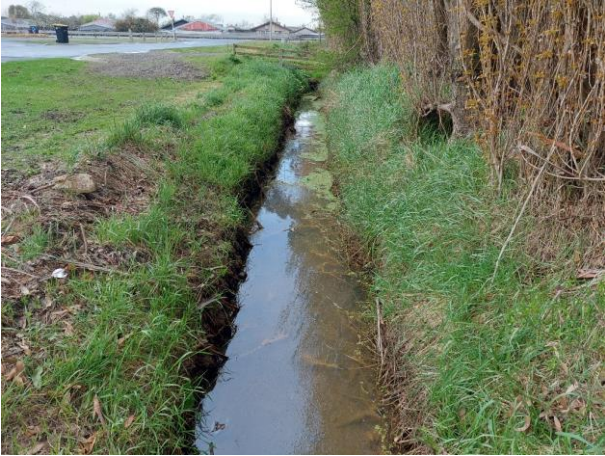
Photo 8: Eastern boundary drain looking downstream to Beach Road
