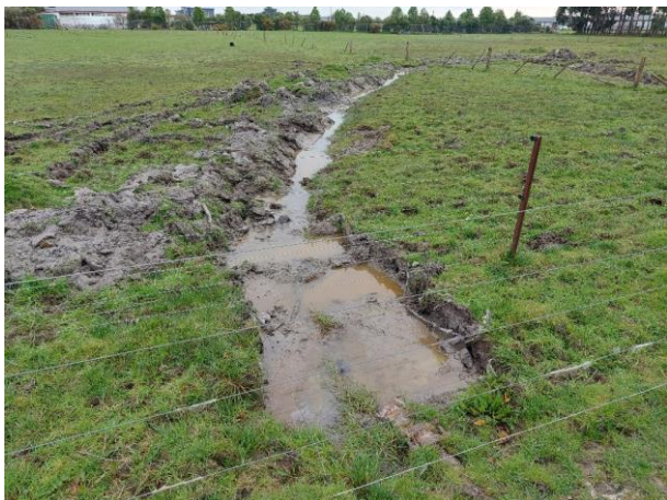
Photo 6: Constructed farm drain
