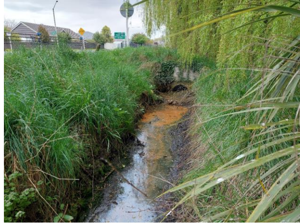
Photo 9: Beach Road drain looking upstream to the culvert
