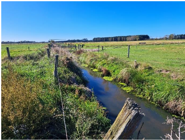
Photo 14: McIntosh Drain looking upstream near the culvert crossing
