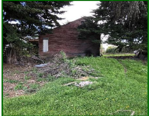
Photo 6 – ACM Super 6 storage area
