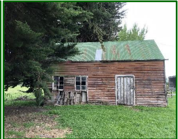
Photo 4 Older farm shed
