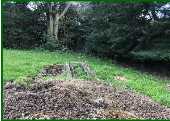
Photo 11 – Concrete trough with burnt material
