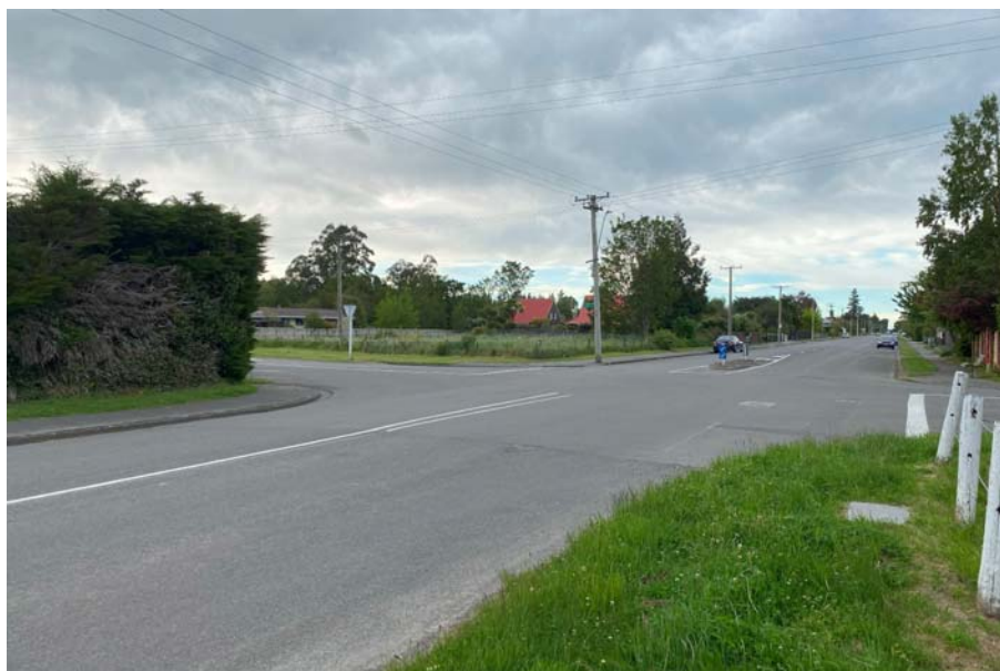
Photograph 5: High Street / Church Street / Weld Street Intersection Looking South
