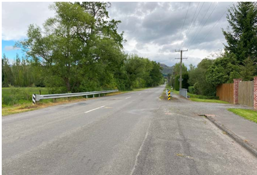
Photograph 3: Culvert and Parking Lane on High Street Looking North (Site on Left)
