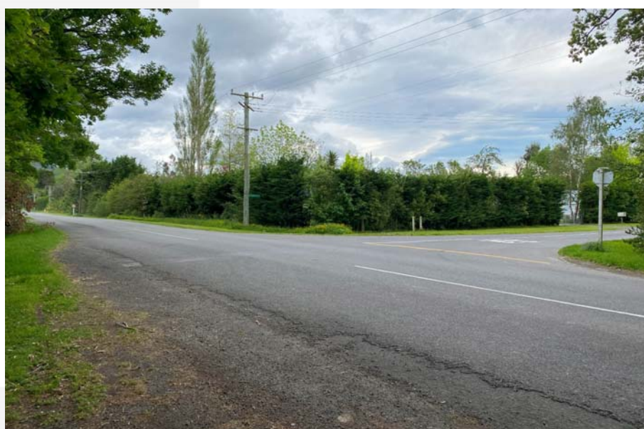
Photograph 2: Ashley Gorge Road / Victoria Street Intersection Looking North
