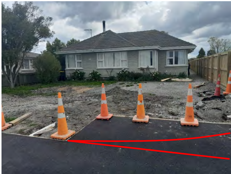
FIGURE 5555 - FRONT OF 67 OTAKI STREET FOLLOWING CONSTRUCTION
