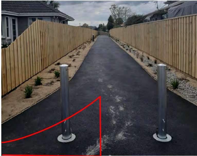
FIGURE 4444 - ACCESSWAY FOLLOWING CONSTRUCTION.
